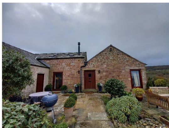
The main entrance route from the drive passes various patio areas and is not well defined.
