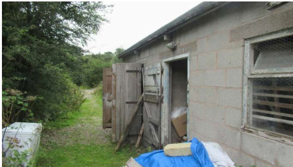
Existing redundant stable block
