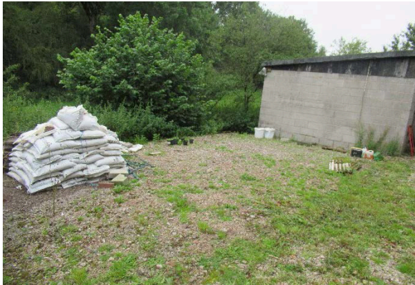
Demolished Garage base & Gable End of Barn
