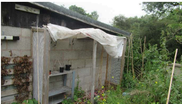
Dwarf wall on remains of goat shed & stable Gable End
