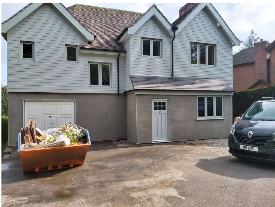
Figure 2 – The dwelling following completion of the works.
