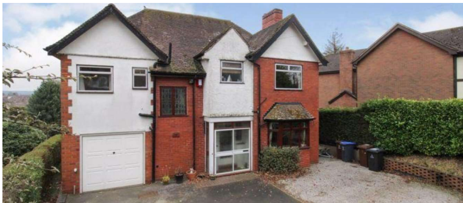
Figure 1 – The dwelling prior to works being carried out
