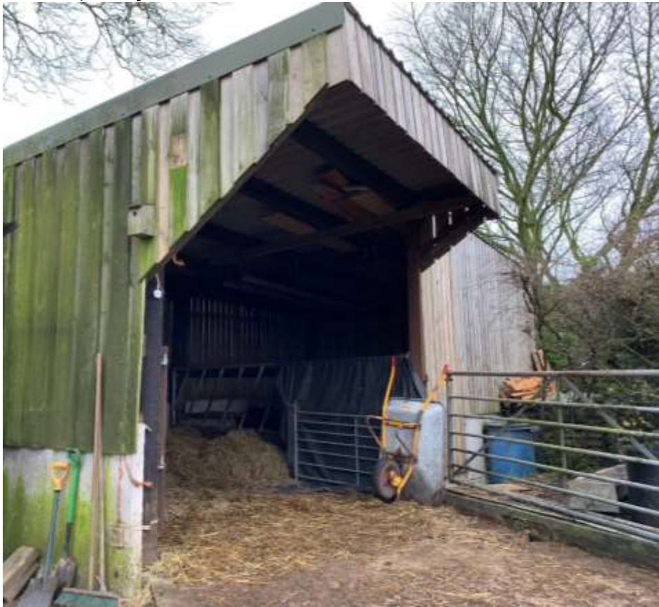
2. Existing Livestock Building
