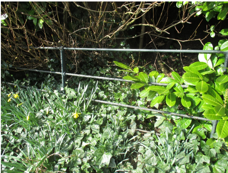
Railing on north side of car park
