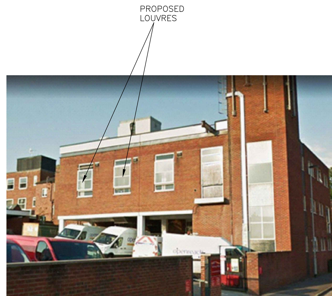
PHOTO OF WEST ELEVATION
