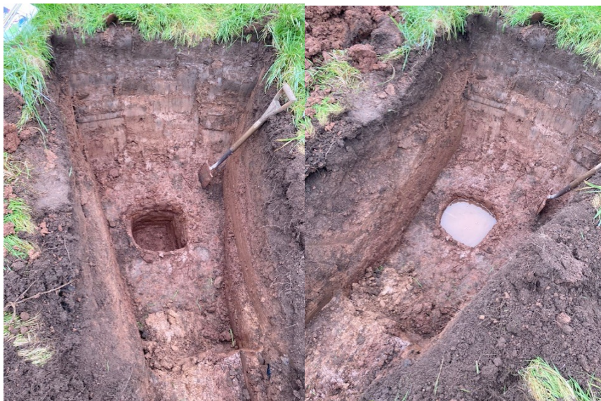
Trail Pit 1 850mm below surface; Before and After Test – water level did not drop
