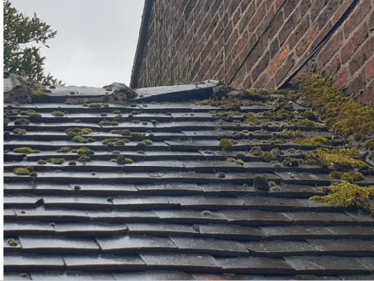
Plate VII. Raised ridge tile on single storey section of farmhouse.
