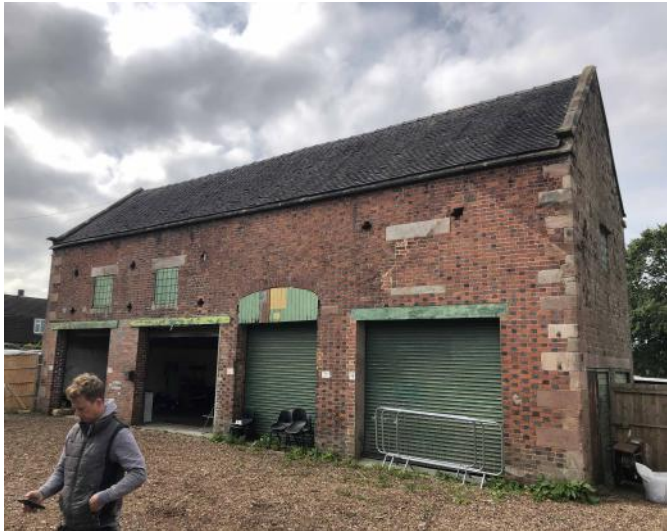
View 6: West Barn
