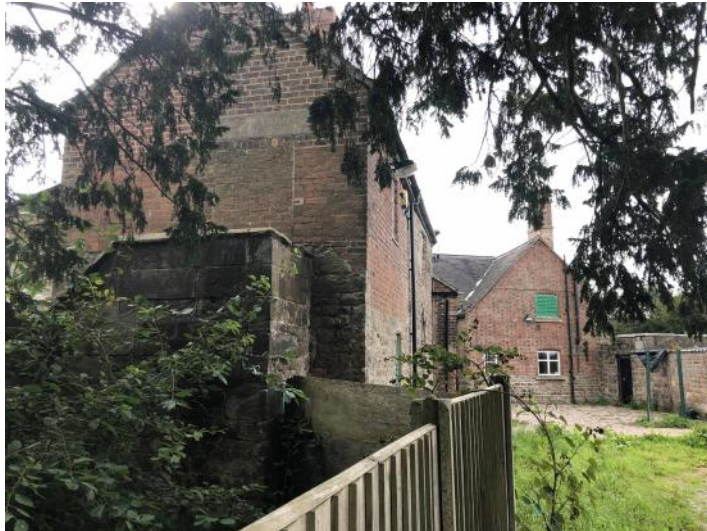
View 8: The North Range Gable
