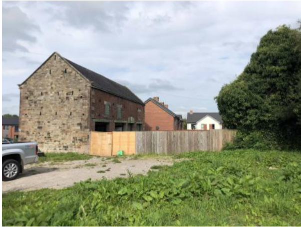
View 2: West Barn
