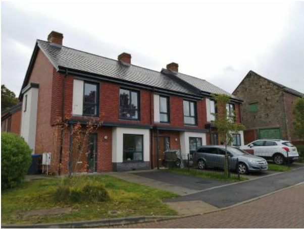
View 4: West Barn from 17-19 Ospray Close
