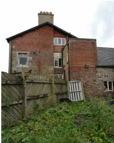
View 13: West Barn from Ospray Close
