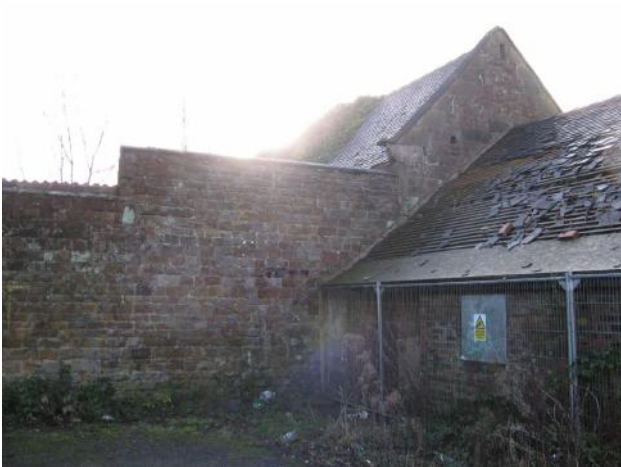
View 11: Haregate Hall North West view
