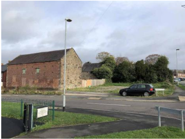
View 1: West Barn from Ospray Close Park
