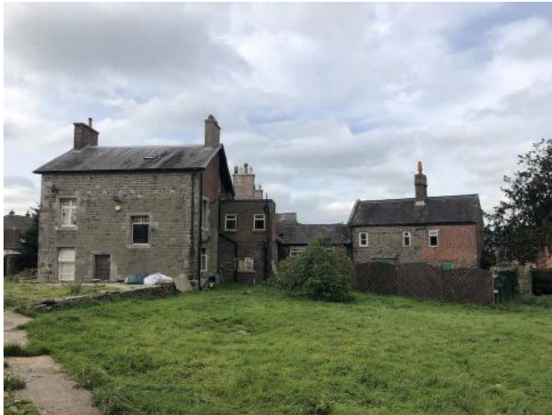
View 12: Haregate Hall North West view
