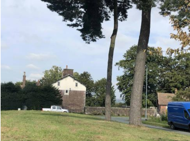
View 15: East Wing Gable End from Queens Drive
