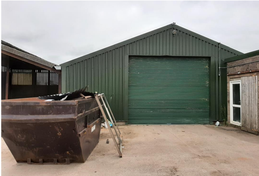
Plate Two: Existing former agricultural outbuildings at Bird Grove Farm
