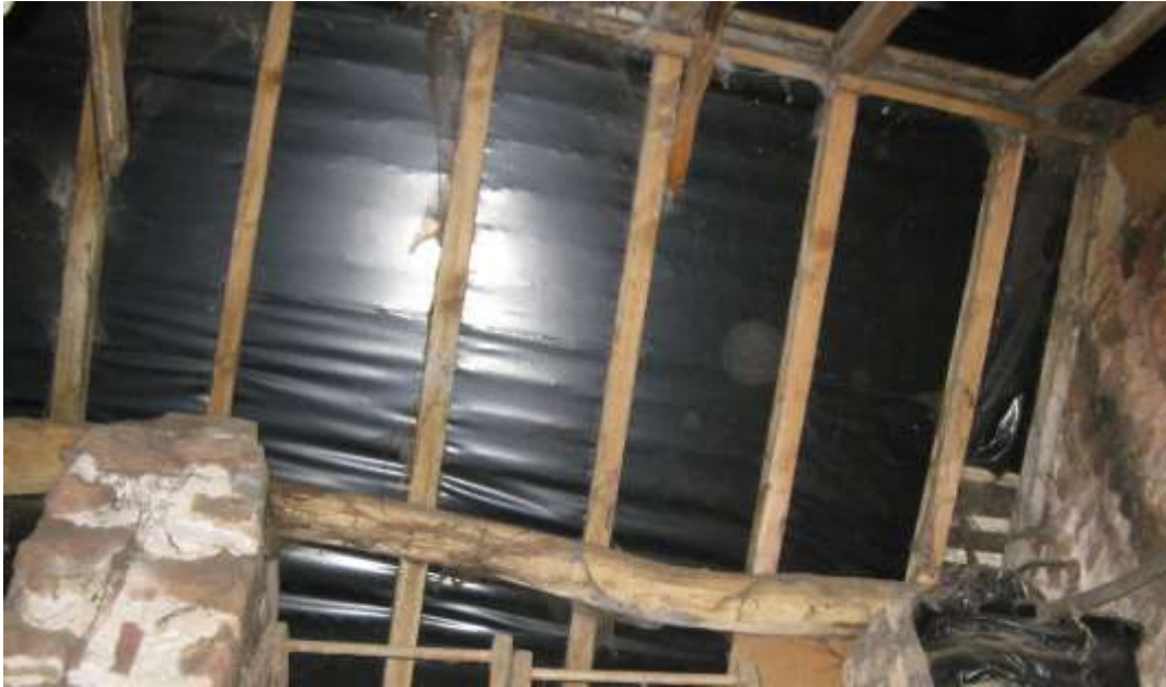
Fig 1.8 Exposed roofing timbers to 2 storey barn (IAA photo 01.10.2020)
