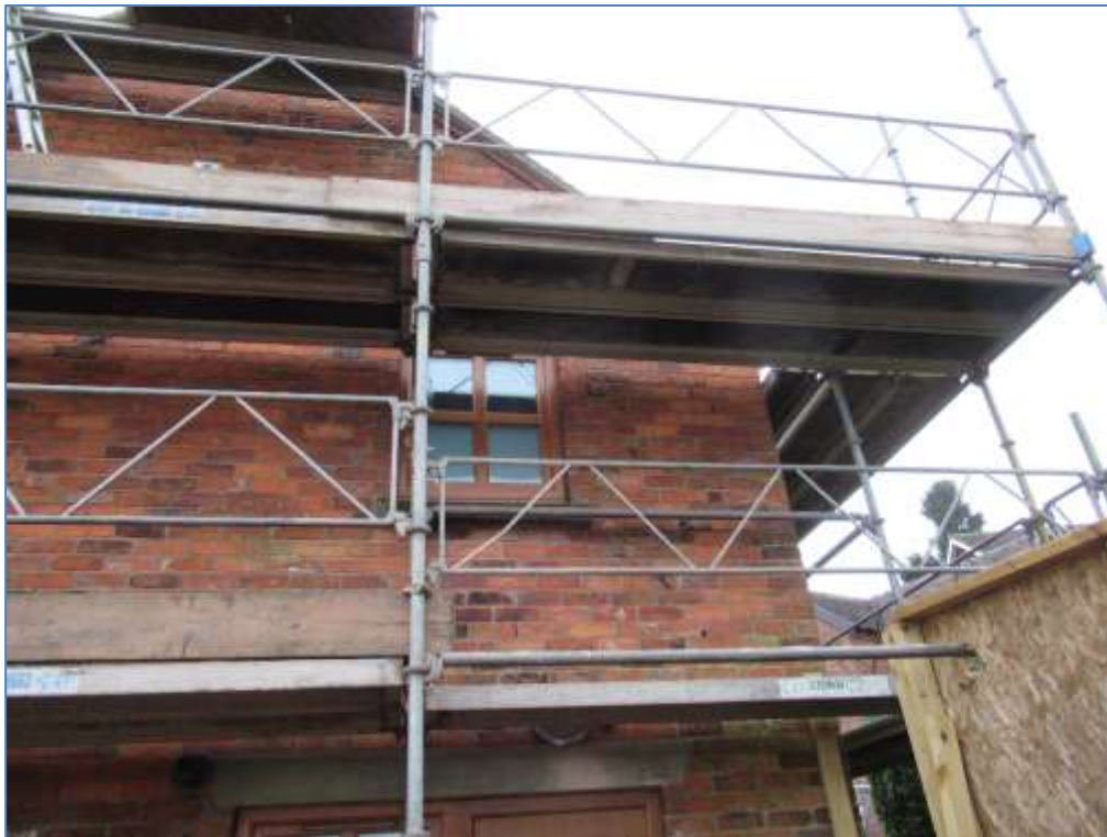
13. View of the upper gable to number 82.
