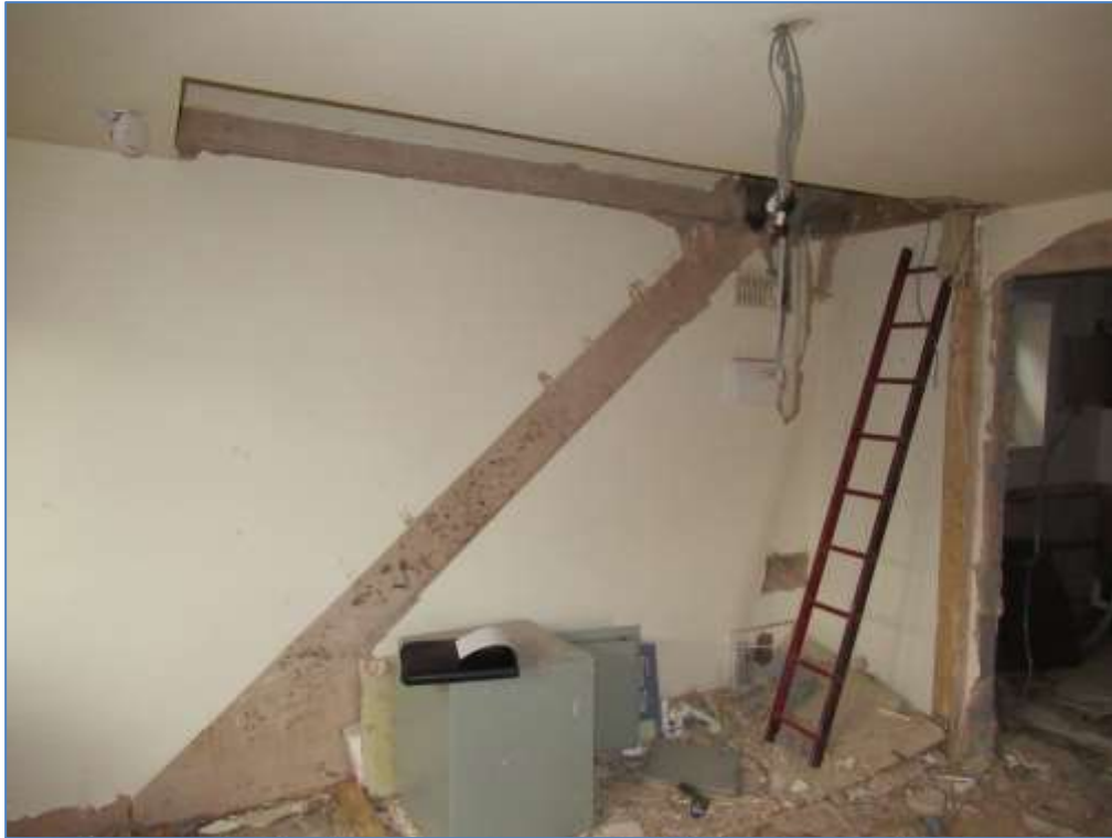
23. Shows area of stairs to number 80.
