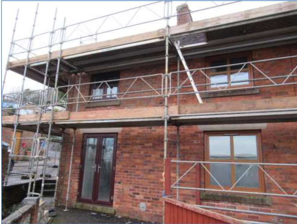
7. General view of the rear of number 80.
