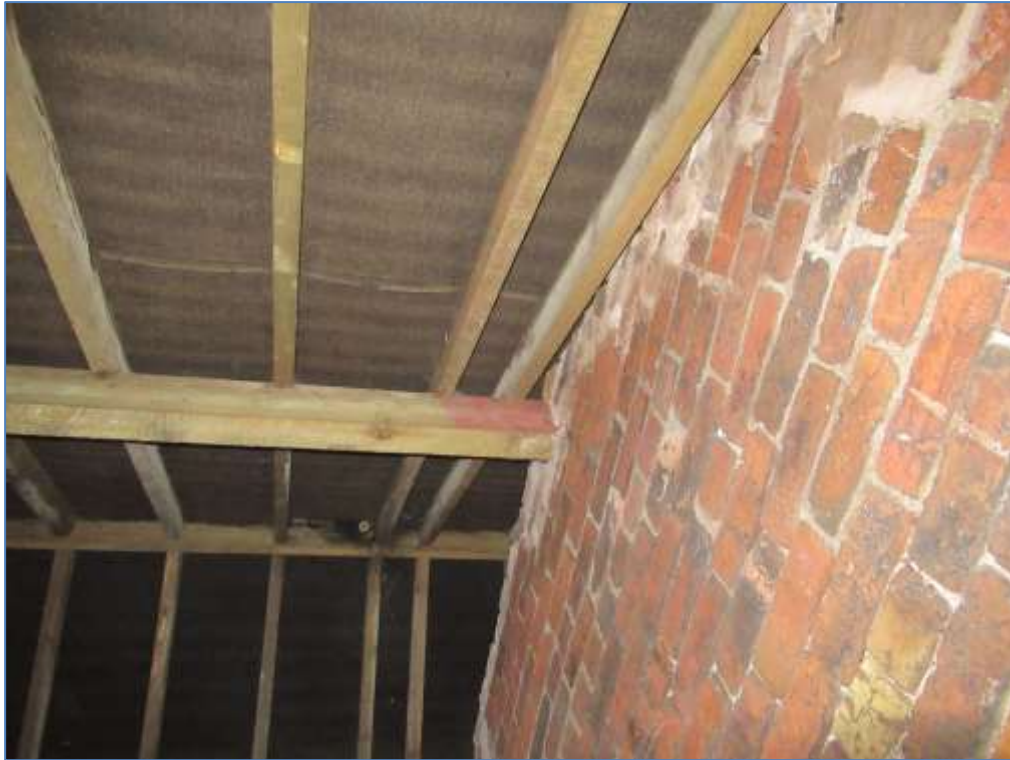
25. Shows modern cut timber roof to the properties.
