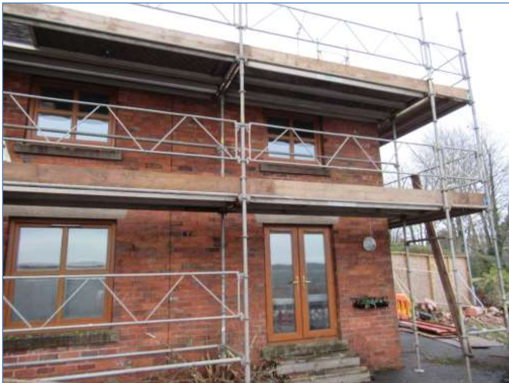
8. General view of the rear of number 82.
