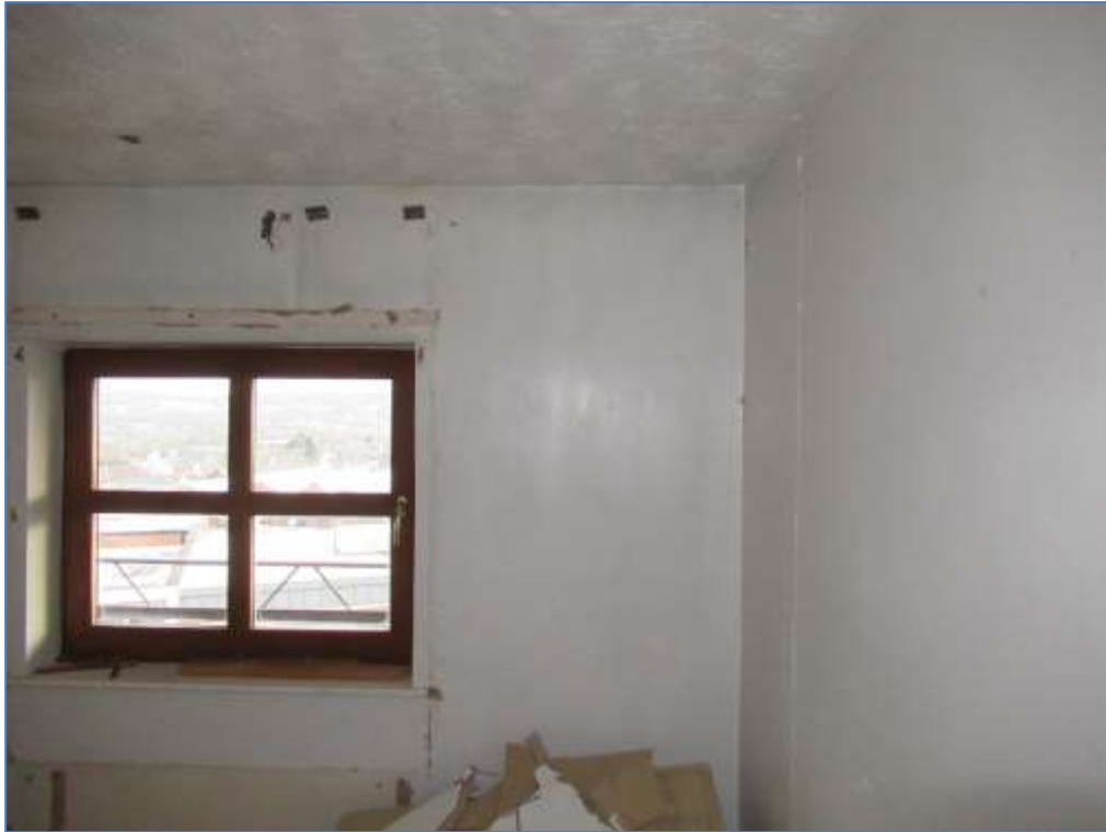
19. View of central bedroom to number 82.
