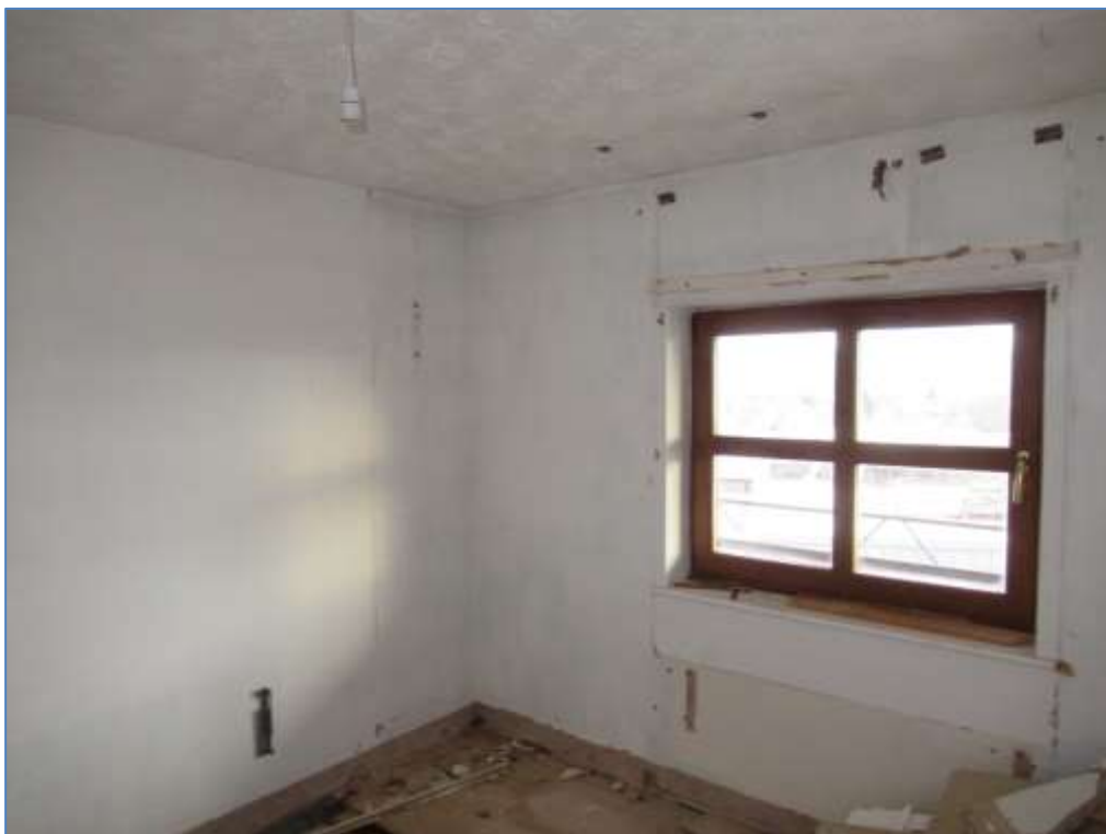
20. View of rear left-hand bedroom to number 82.
