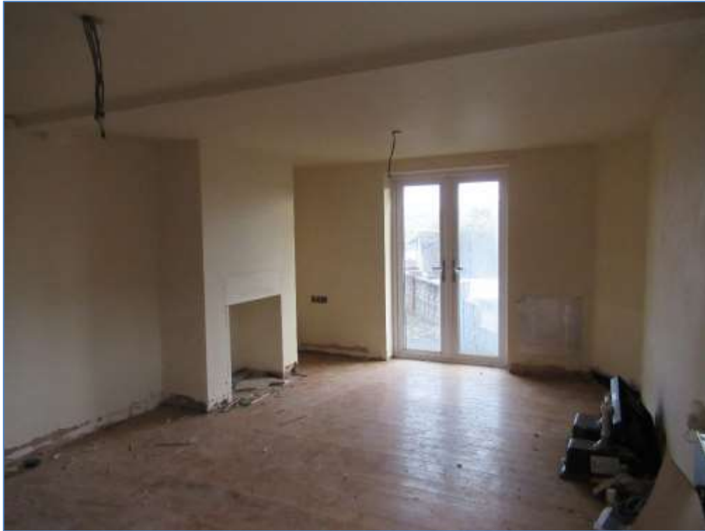
21. View of lounge to number 80 showing patio doors.
