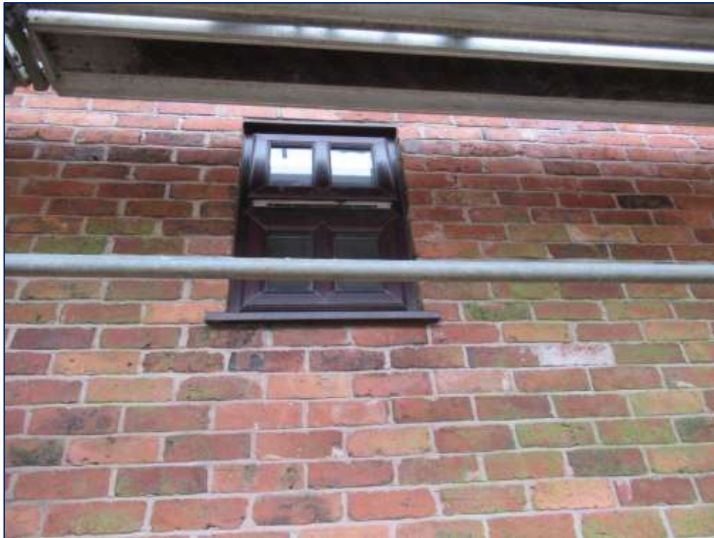
3. View showing the stairwell window to number 80.
