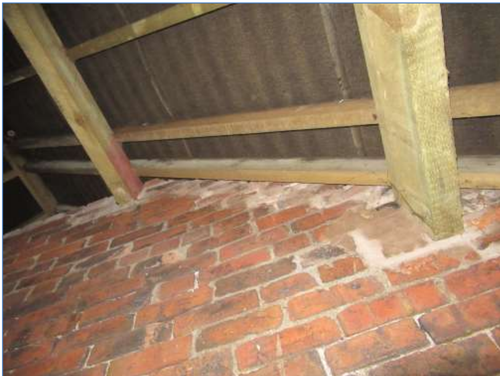
26. Shows modern cut timber roof to the properties.
