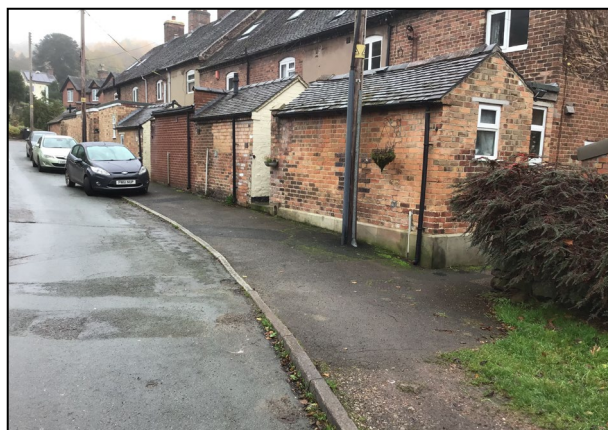
Photo 1 – View of the rear of No's 10-17 The Square
