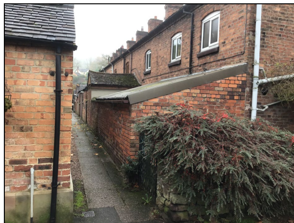
Photo 2 – View of the rear of No's 2-9 The Square
