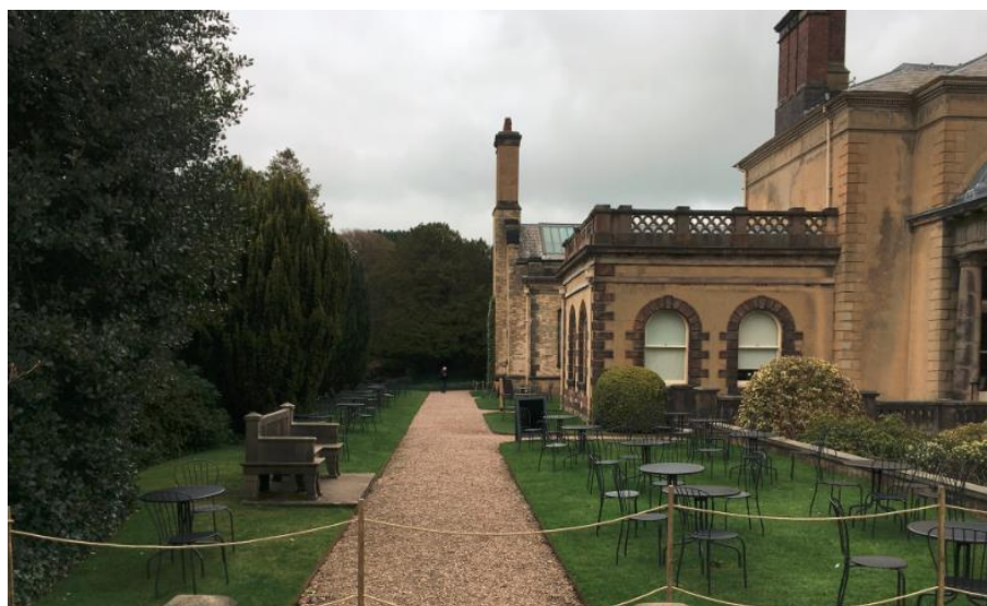
View from the bandstand along the terrace at the west elevation of the house
