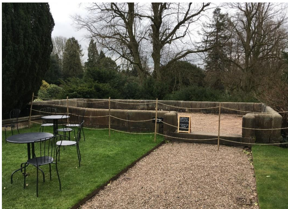
View to the bandstand showing the dense planting to the south & west elevations of the Bandstand
