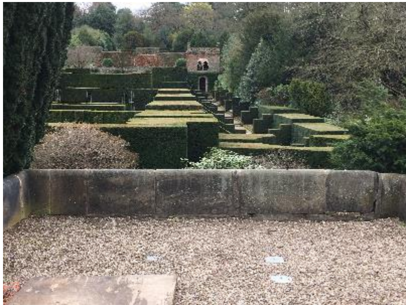
Internal view of East wall of Bandstand
