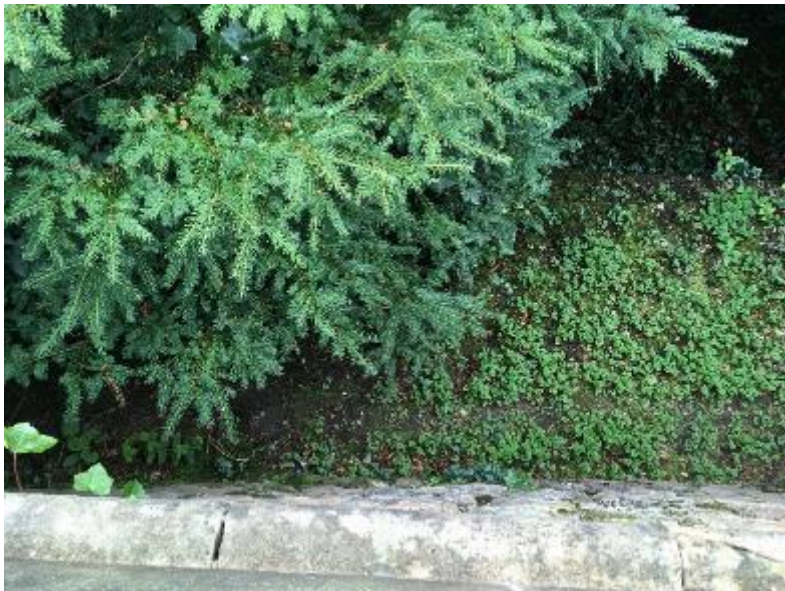
Adjacent South Wall of Bandstand
