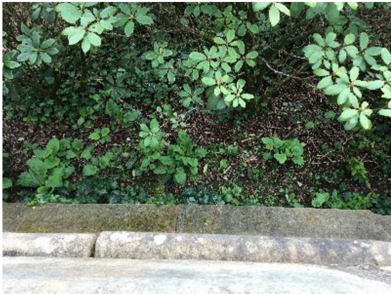
Adjacent East Wall of Bandstand
