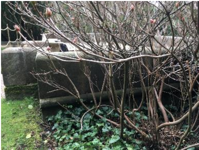
Adjacent West Wall of Bandstand
