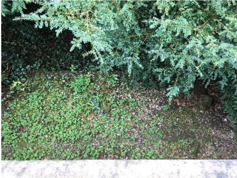
Adjacent South Wall of Bandstand
