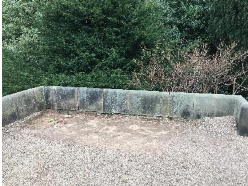
Internal view of West wall of Bandstand
