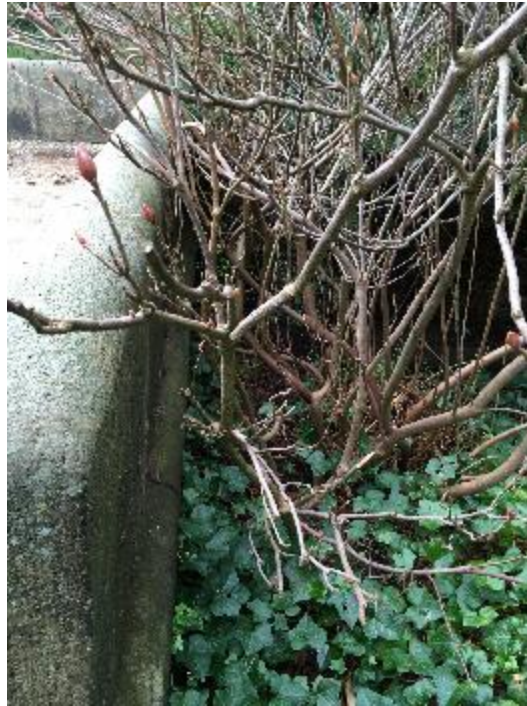
Adjacent West Wall of Bandstand
