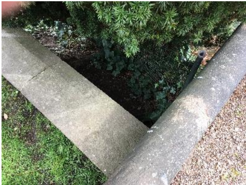
Adjacent North Wall of Bandstand
