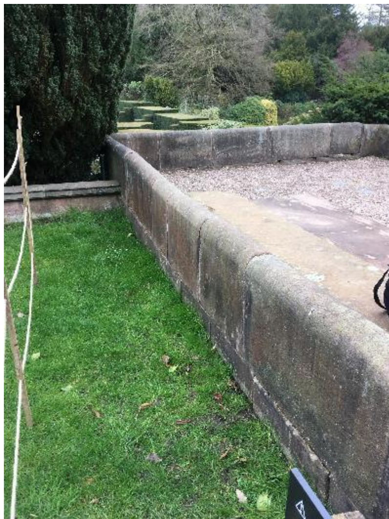
View of North wall of Bandstand
