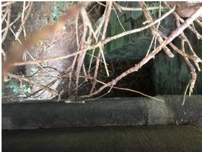
Adjacent West Wall of Bandstand
