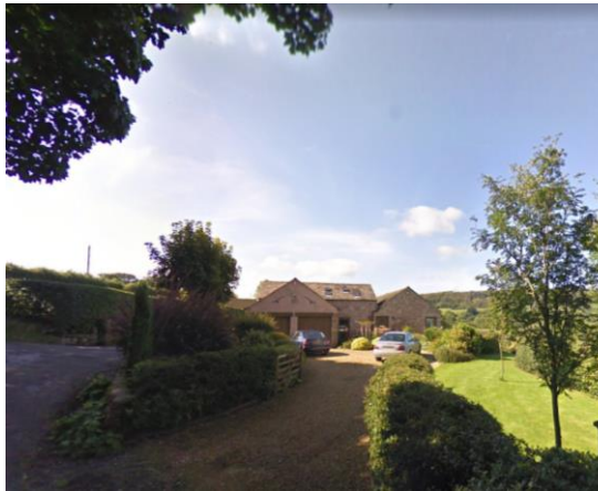
The property is nestled on a sloping site that conceals parts of it from the highway.
