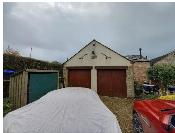
The door openings are too narrow for modern vehicles to manoeuvre in and out of the garage.
