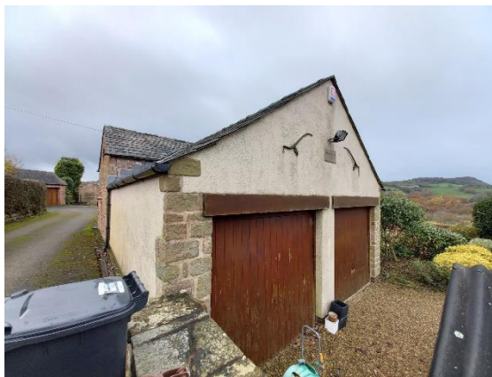
The existing garage is set partially into the sloping site against a neighbour's driveway.
