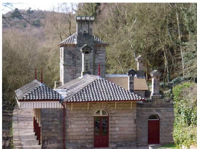
Alton Station viewed from the Farley Lane road bridge
