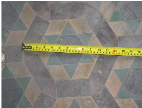
Detail of Waiting Room floor tiling
