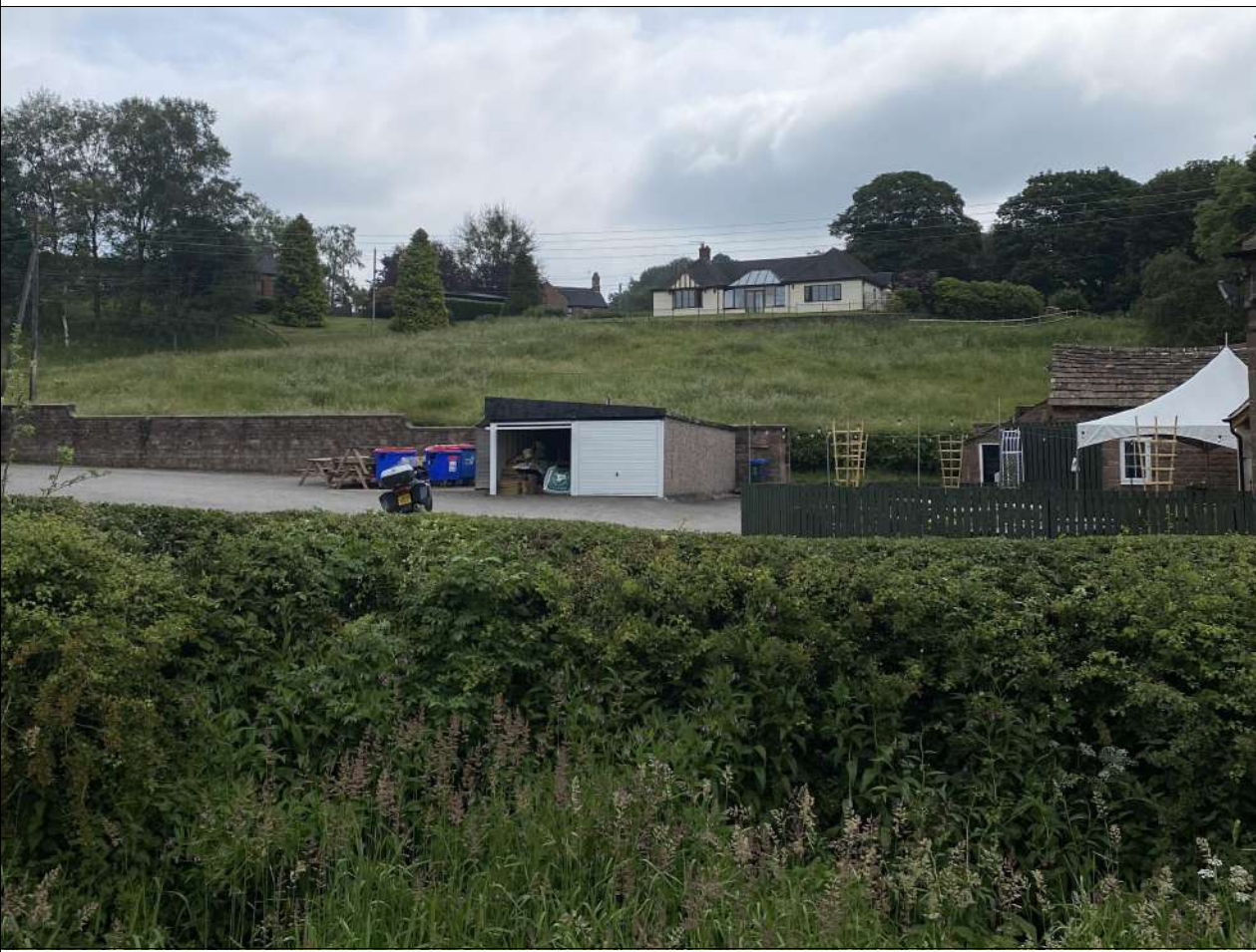
Photo 2: View into development site from A523.
