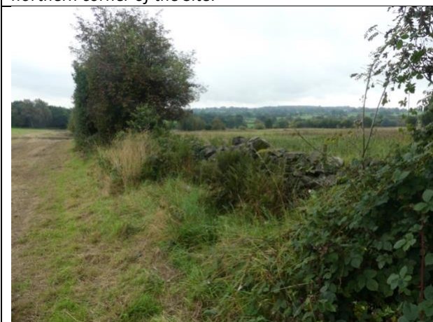
Photo 5: Stone wall, scrub and hedgerow along the south-western boundary.
