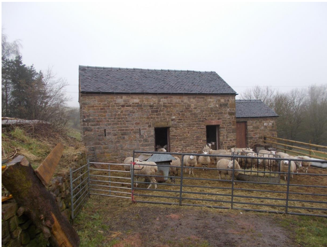
THE BUILDING FROM THE SOUTH EAST
