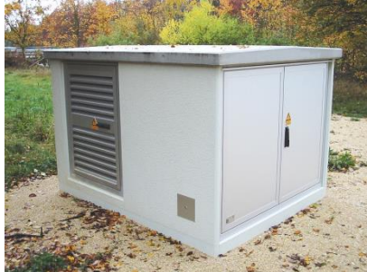
Figure 5. Example of a 20 kV / 400 kV transformer station.
