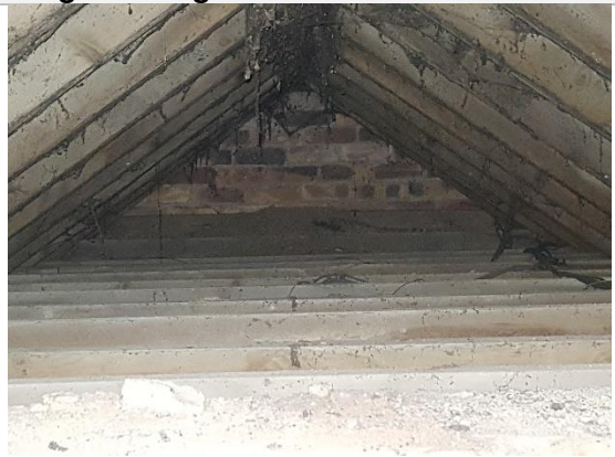
Plate X. Roof void looking southward with no division.
