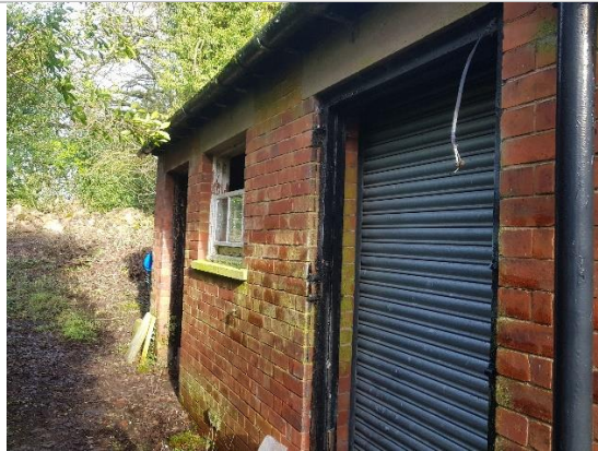
Plate III. Roller shutters and open window and door along the western elevation.
