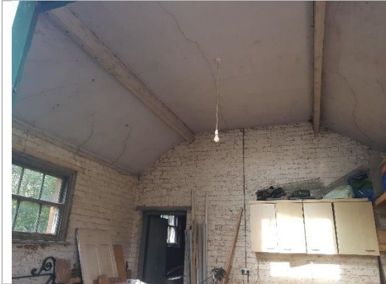
Plate VII. Southern room with bare brick walls and plastered lath ceiling.
