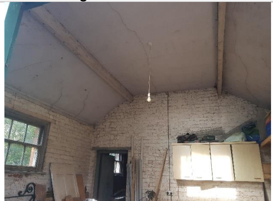
Plate VI. Southern room with bare brick walls and plastered lath ceiling.
