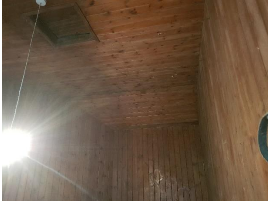
Plate VII. Second room clad in pine tongue and groove boards
