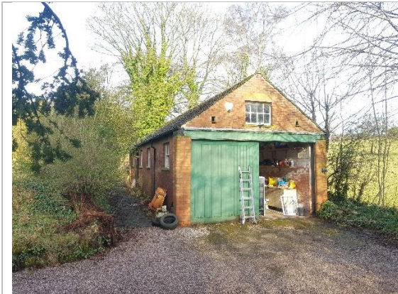
Plate I. Southern elevation with sliding doors and pigeon holes in masonry above.
