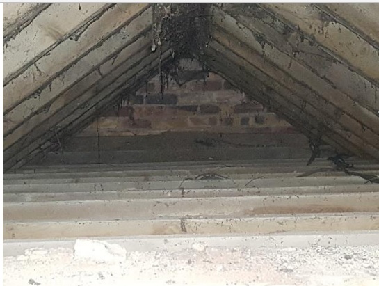
Plate IX. Roof void looking southward with no division.
