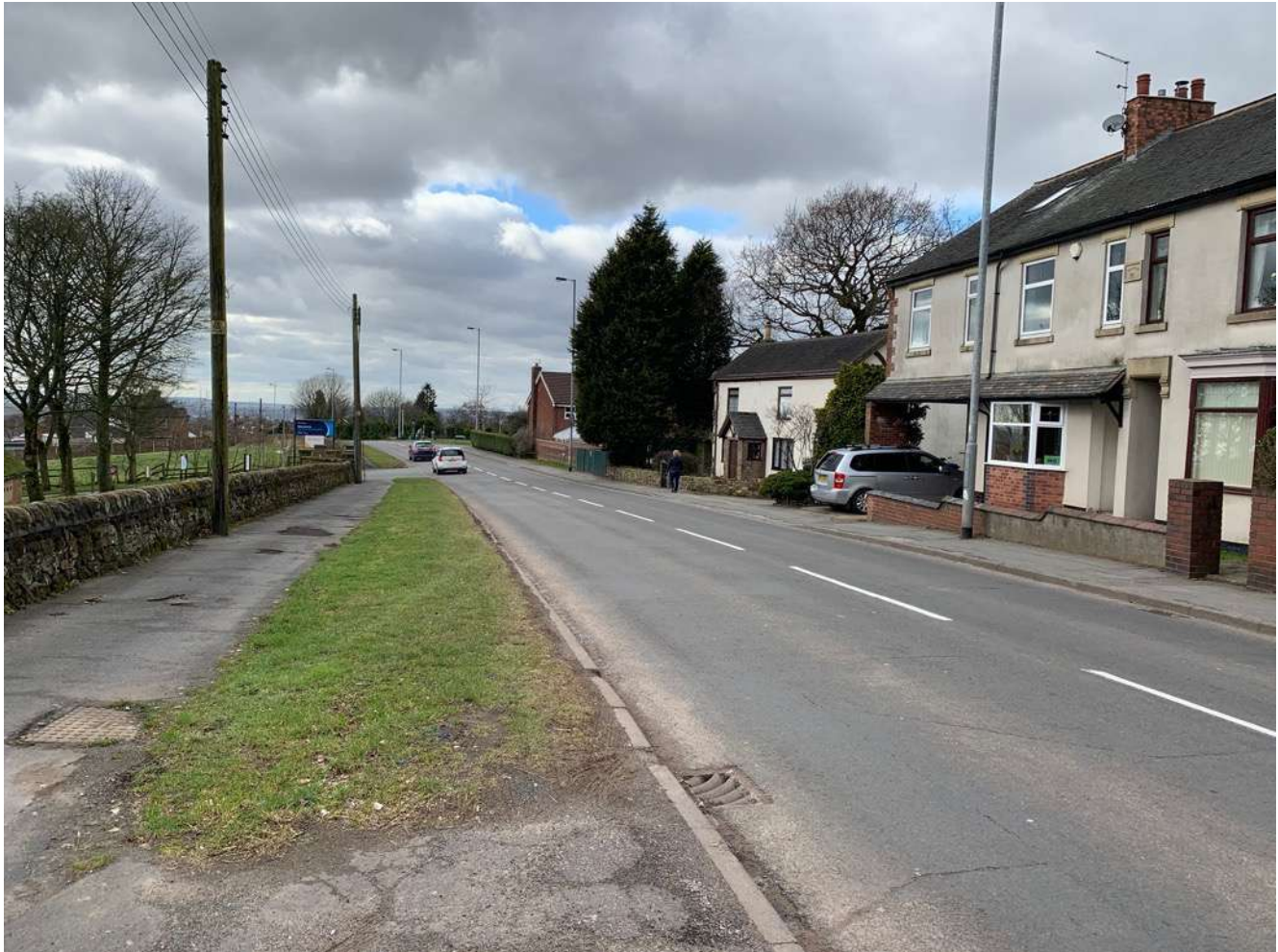
Figure 3.2: Ash Bank Road – Westbound
