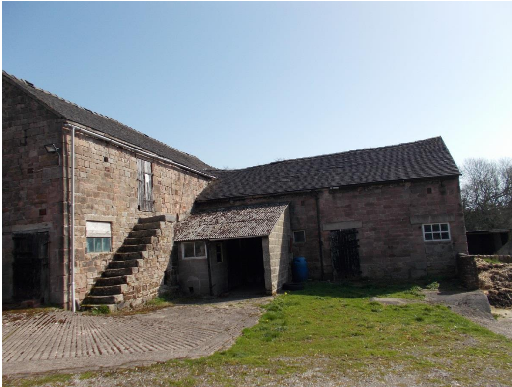
WEST END OF BARN 1 AND WEST ELEVATION TO BARN 2
