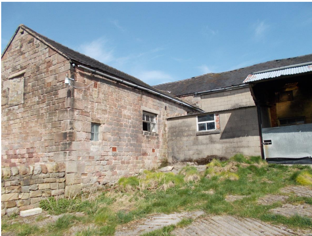
END OF BARN 2 AND EASTERN SOUTH FACING PART OF BARN 1
