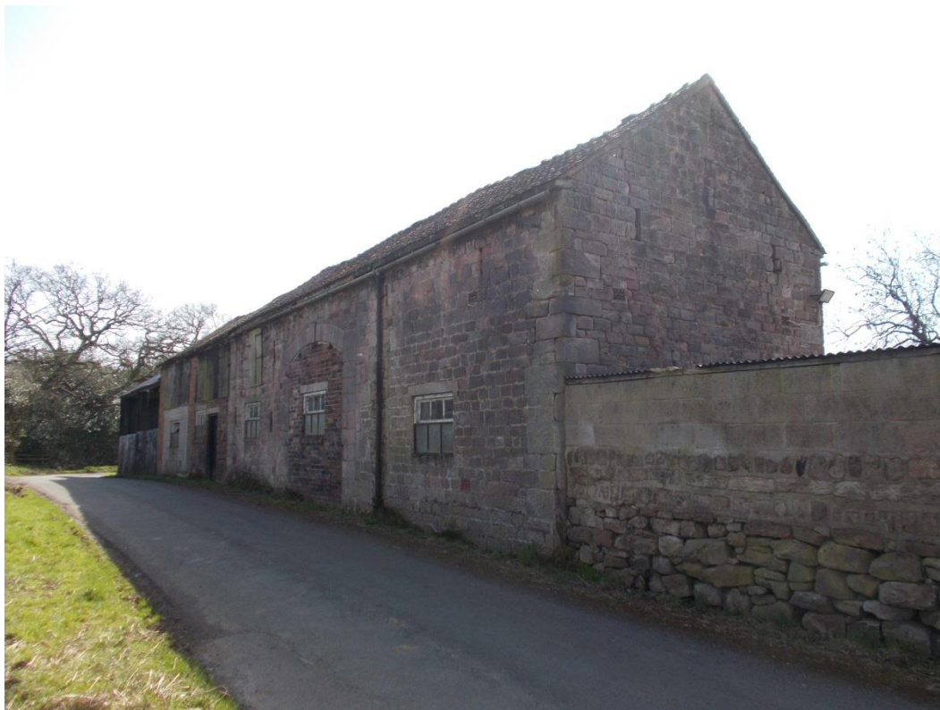
BARN 1 from the west showing road frontage: note infilling of former hay waggon opening and concrete block infilling of eastern end hay barn
