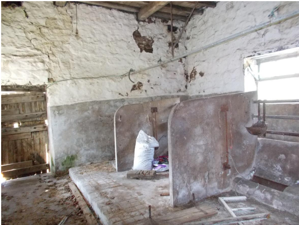
INTERNAL OF BARN 1 WESTERN END showing boskins, feed troughs, heel stones, muck passage etc.
