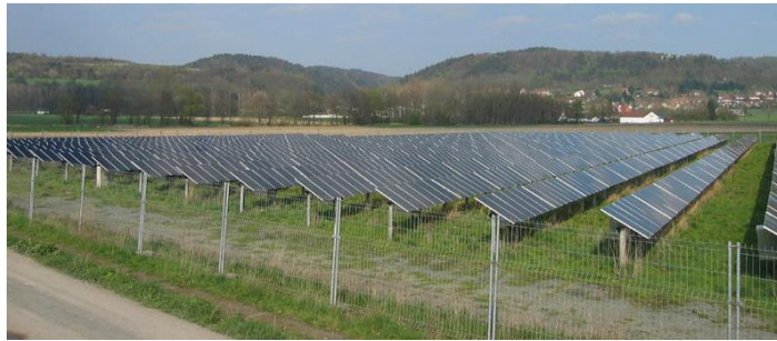
Figure 2. Module tables oriented towards the south.
