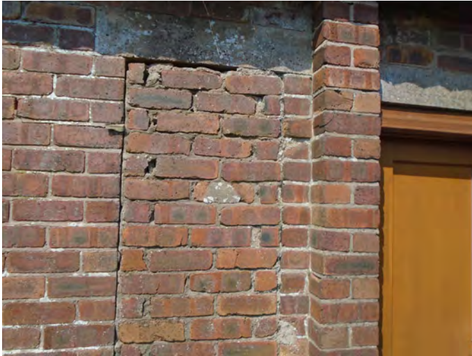
Building A. Infilled window detail - typical of all buildings.
