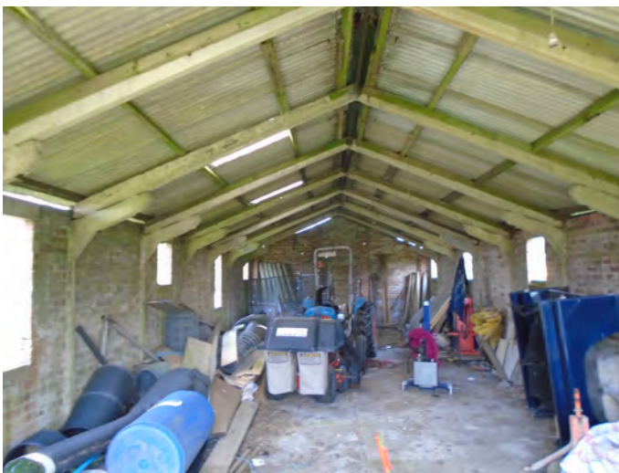
Building D. Internal view.
