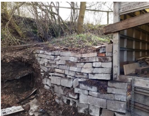
Fig 10: The base of T6 on higher ground
