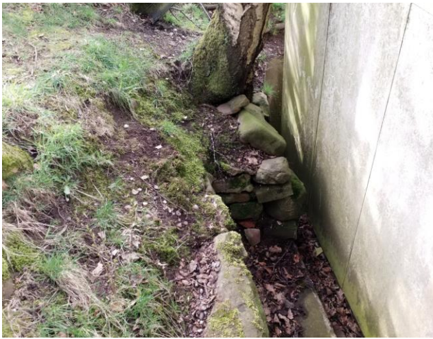
Fig 4: The base of T1, on top of a retaining wall
