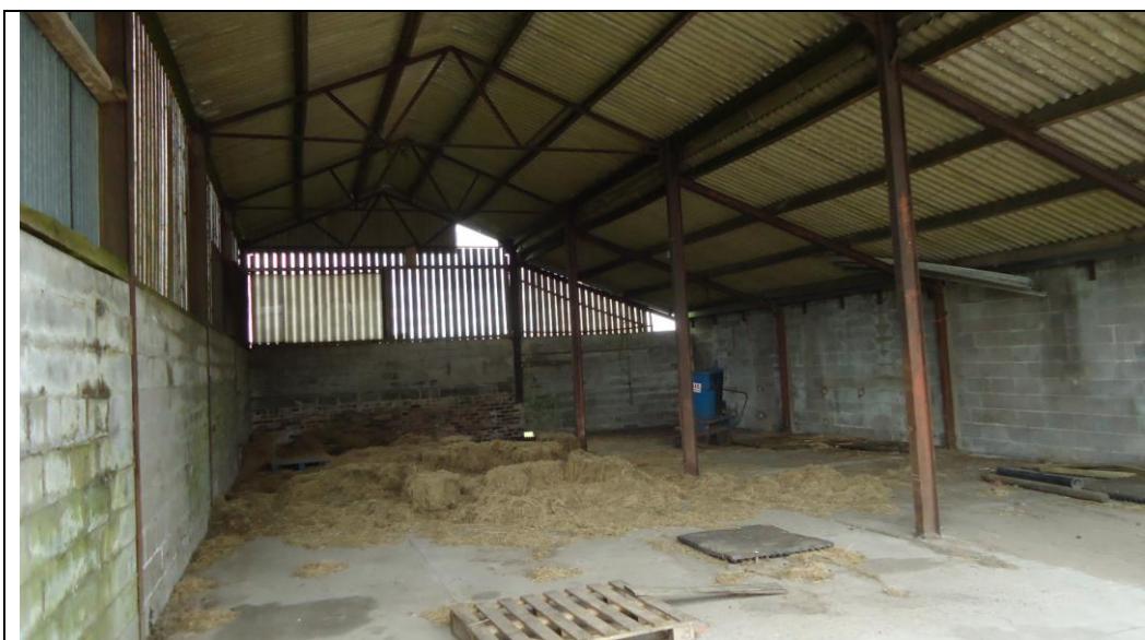
Plate 5: Interior of existing building (TN3)
