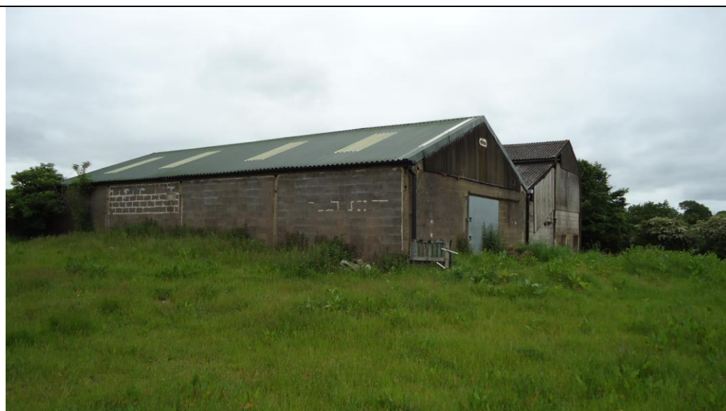
Plate 6: Looking at the north and eastern elevations of the existing buildings on site (TN3)
