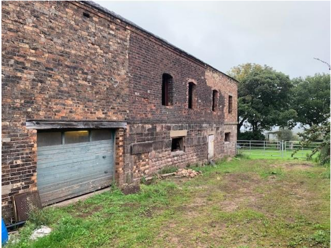
External view of south east barn showing stonework at ground floor level and brick work masonry at first floor.
