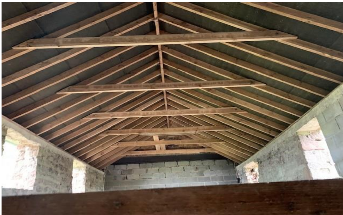
General view of relatively new roof to north east section, will require some minor strengthening for domestic conversion.
