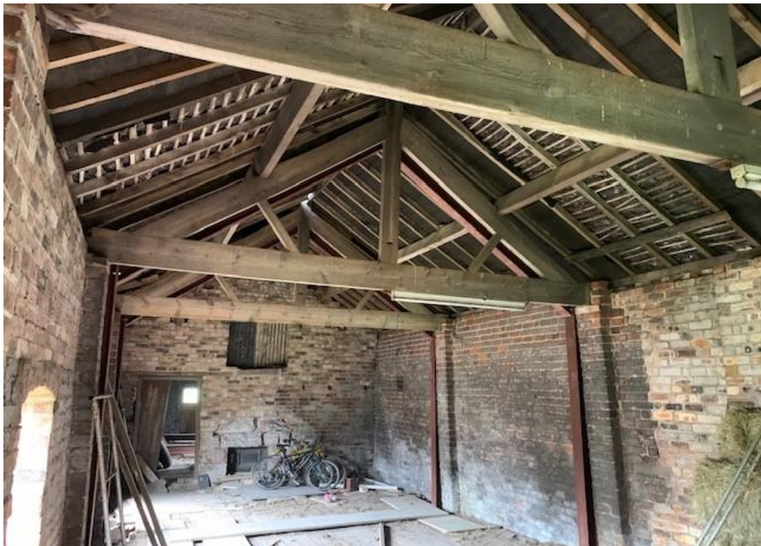
Another internal first floor view of north east section – note timber trusses, purlins and rafters generally in good condition.
