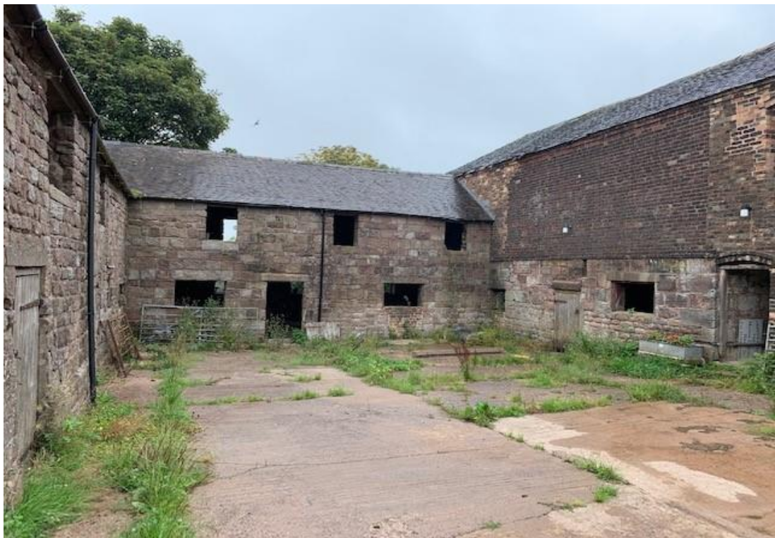
Stone work and roof of north east section in good condition.
