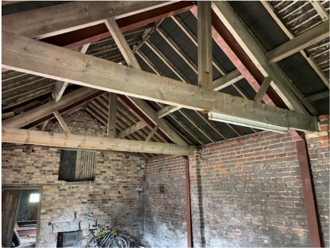
Typical internal view of first floor south east section – note previously installed steel portal frames providing lateral stability.
