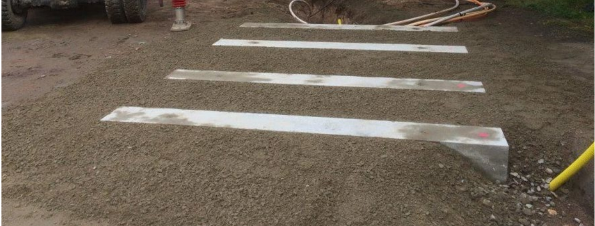
Photograph 2: Shelter foundations
