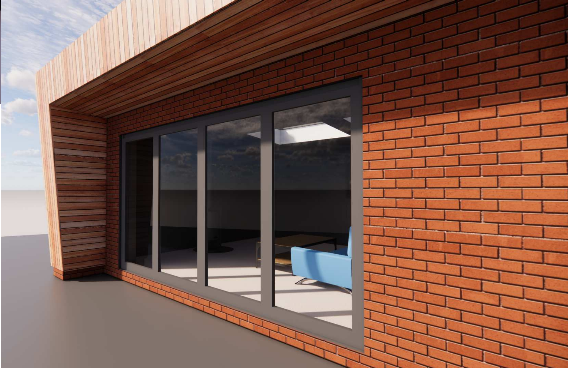
External - Close-up to Leaning Facade & Red Western Cedar Cladding
