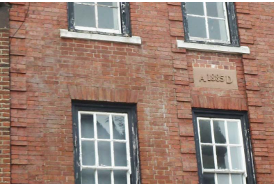
2. Ibstock Old English Birtley (eg. Rusticated Brickwork, Leek)
