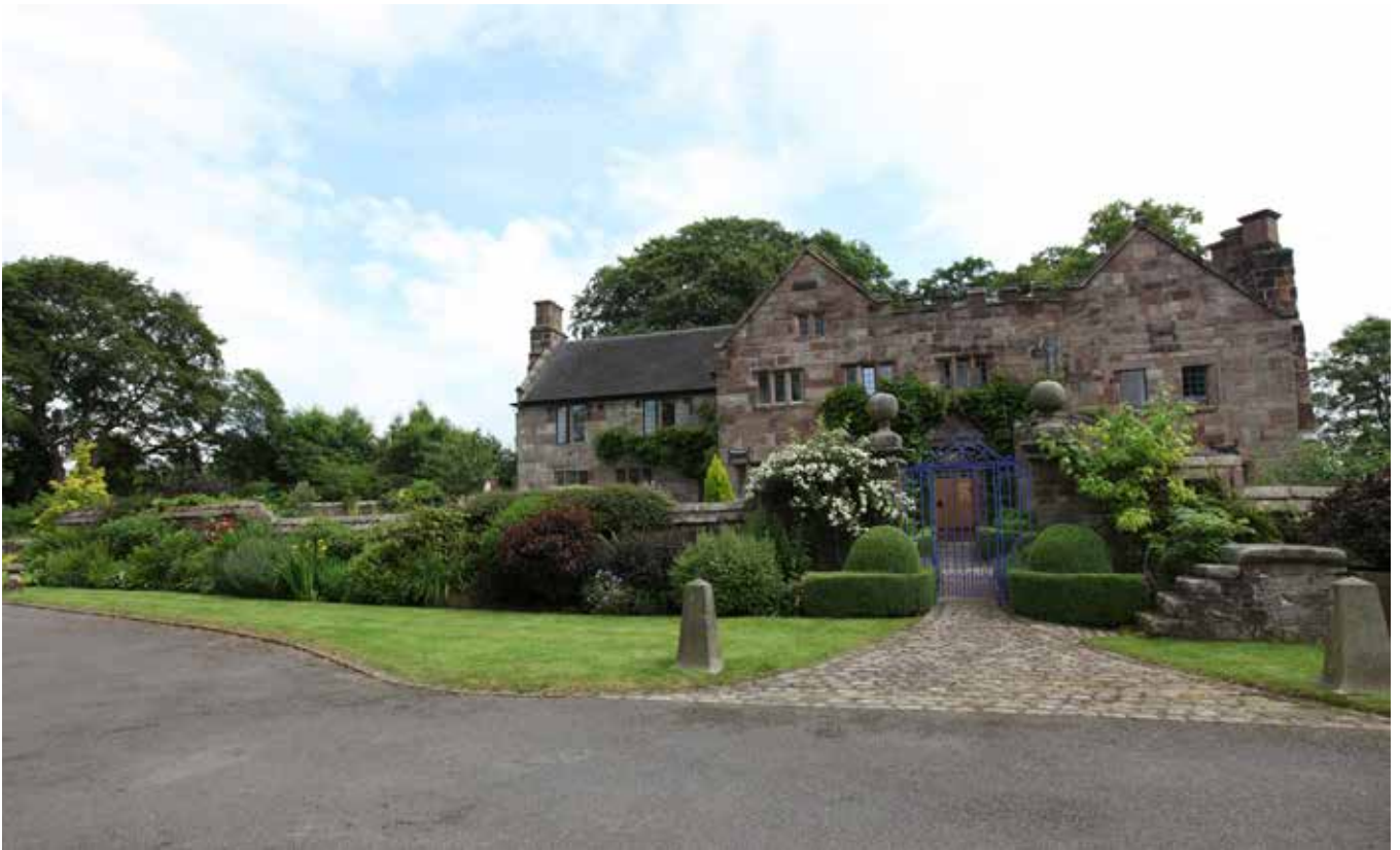
16. Front / south elevation of Stonelowe Hall, as seen from the converged footpath network. The walled enclosed garden 'court' to the front of the building has been lowered at some point to enable outward views. As a result, there will be glimpsed views only of the parapet of the Orangery.
