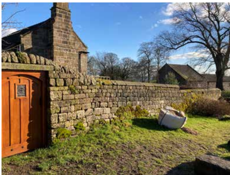
3 View of the western wall behind the house, from public footpath Longsdon with rebuilt section around the gate (Stonelowe Hall - 2021).
