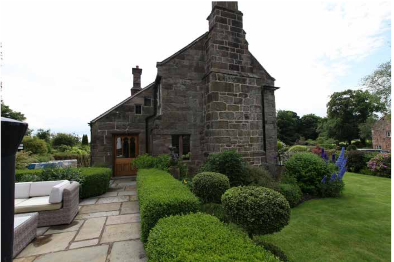
18. Elevation of the western gable with its mass masonry external stack. The masonry stack and surrounding stonework on this elevation is sensitive to change; an extension here, whether a link or a wing, would harm the listed building. The proposed structure is completely detached from the listed building and would not harm the significance of the listed building or its setting.
