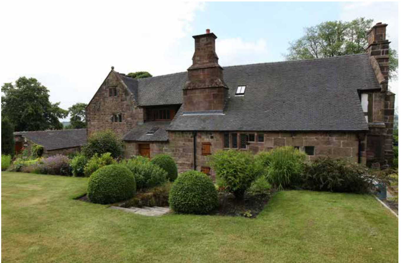
20. Rear elevation of the listed building. The simple massing of the catslide roof, and the massing of the one enclosed (formerly external) large masonry stack have the greatest impacts, whilst the masonry and exposed timber-frame reveals a plethora of changes to the building over time - a long period of evolution and change to a large and important historic building.
