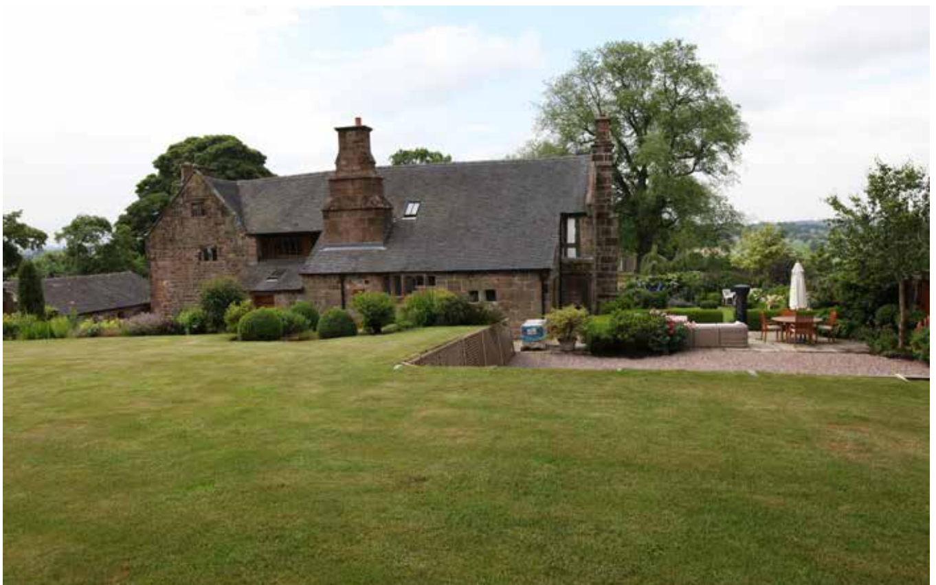
21. View of the rear of the listed building from the north lawn. The large area of lawn and simple treatment in this view echoes the large expanse of clay tiled roof. From this angle, the new Orangery will have a low impact, as the new lawn will rise gradually to a green roof and will read as a continuation of the existing lawn. It will not affect how we appreciate the main listed building.
