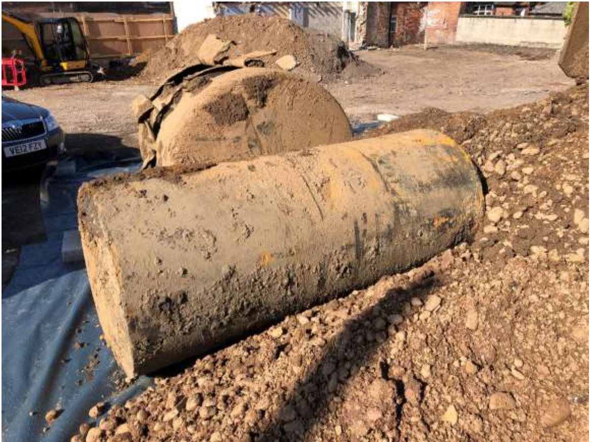
Photo 1: Excavated Tanks (Tank 1 at back)
