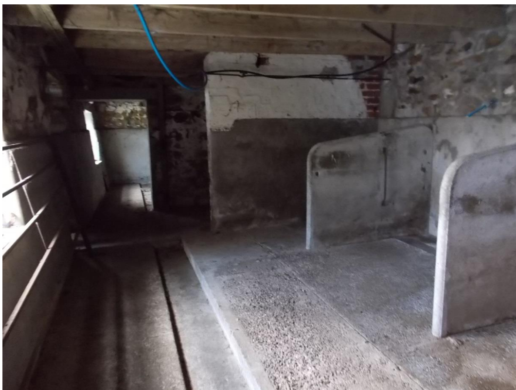
INTERNAL OF THE TWO STOREY BARN SHOWING BOSKINS, HEEL STONE AND MUCK PASSAGE
