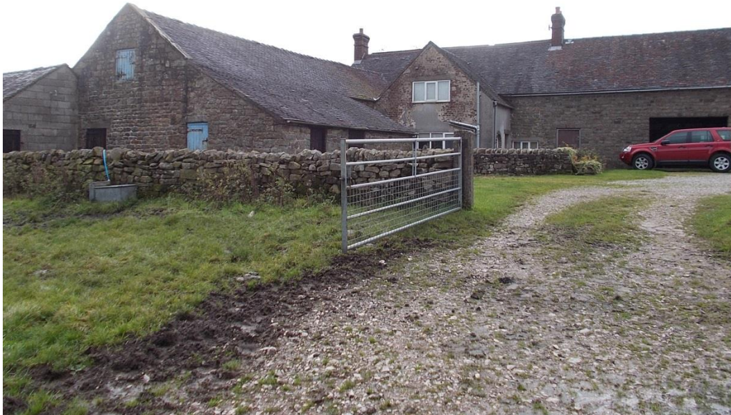
THE TWO STOREY PART TO BE CONVERTED WITH ATTACHED FARMHOUSE BEYOND WITH YARD PARKING – VIEW FROM NORTH EAST
