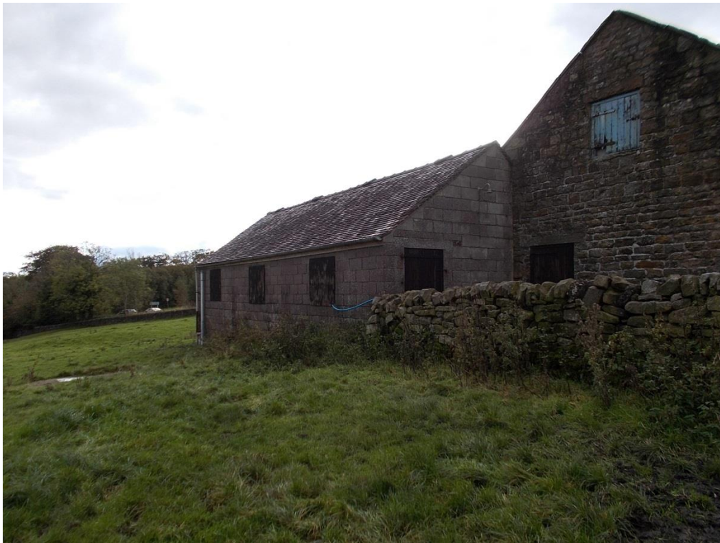
VIEW FROM NORTH EAST SHOWING THE GABLE END OF THE TWO STOREY BARN AND THE SINGLE STOREY ATTACHED BUILDING
