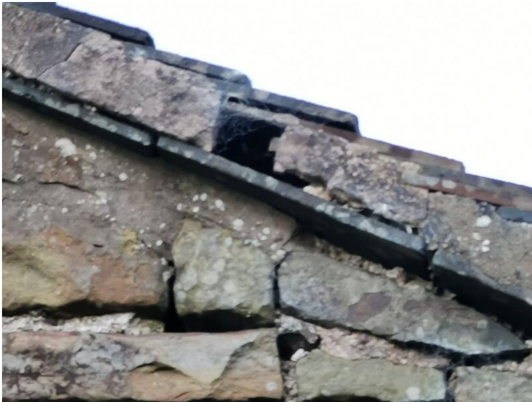
Plate 3: A photograph showing the missing mortar between the stone work.
