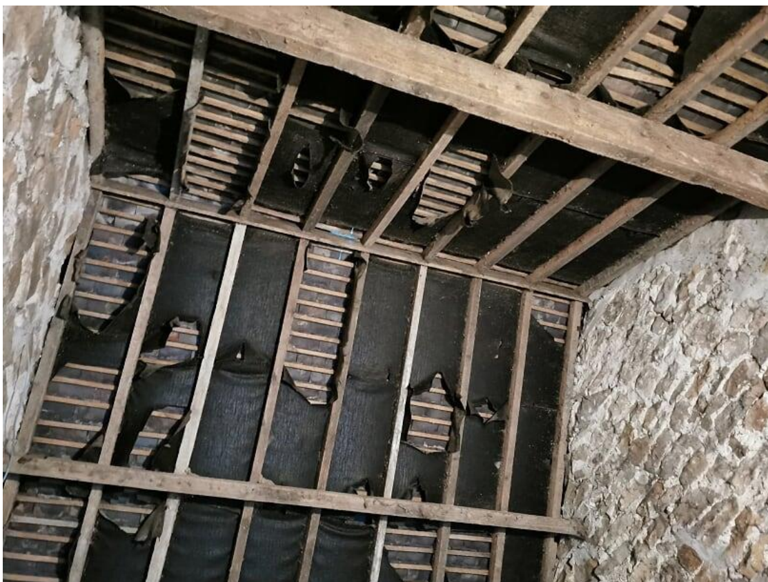
Plate 5: A photograph of the internal of the surveyed barn showing the membrane under the tiles.
