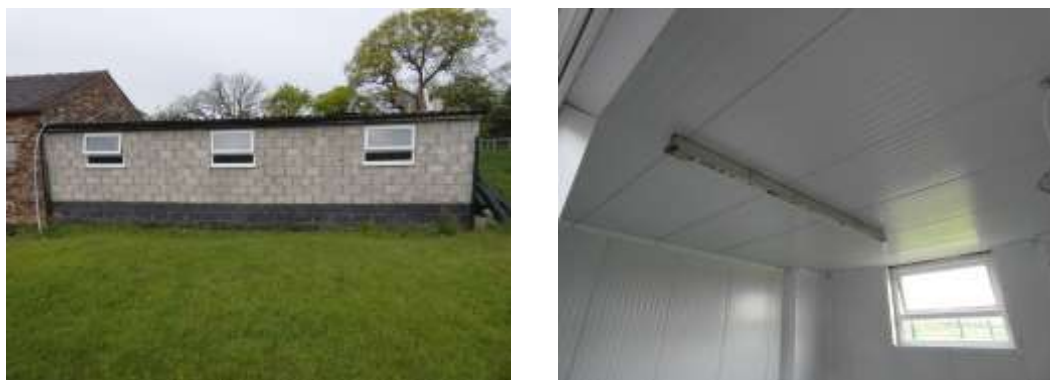
Figs. 21 and 22 Exterior and interior of kennels
