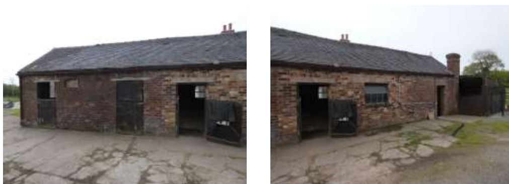
Figs. 7 & 8 Roof of the brick built stables
