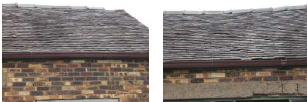
Figs. 15 & 16 Roof of the barn
