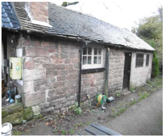
West side elevation with showing original and rebuilt stone walls
