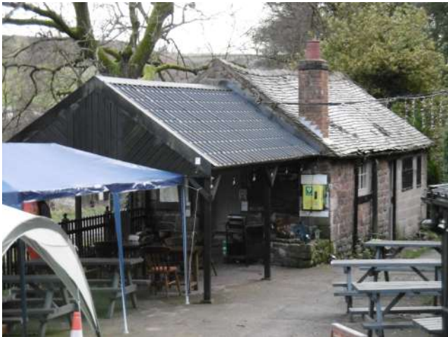
North elevation showing roof undulations and veranda
