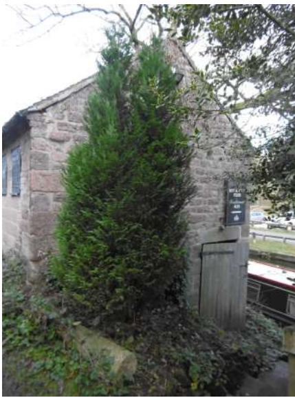
South gable wall with basement entrance alongside canal
