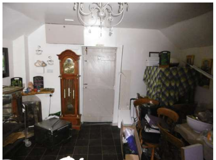
Internal view of north gable dry lined cafe walls
