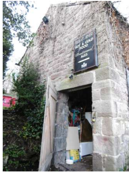
South gable with entrance to basement at canal side
