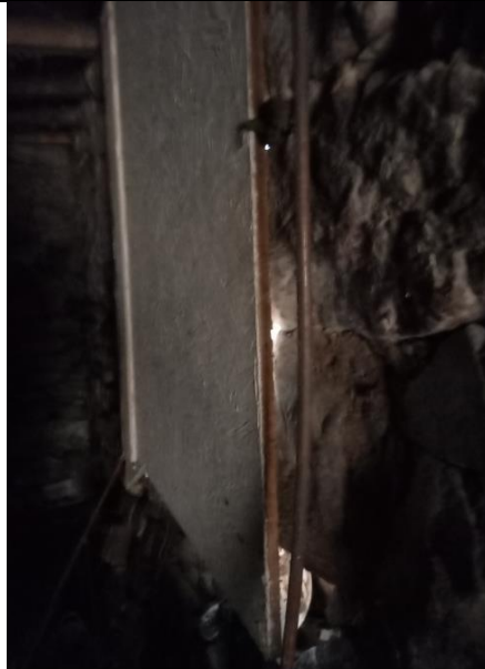
Plate 13: Photograph showing the light coming through the boarded window. Photograph facing north-east.
