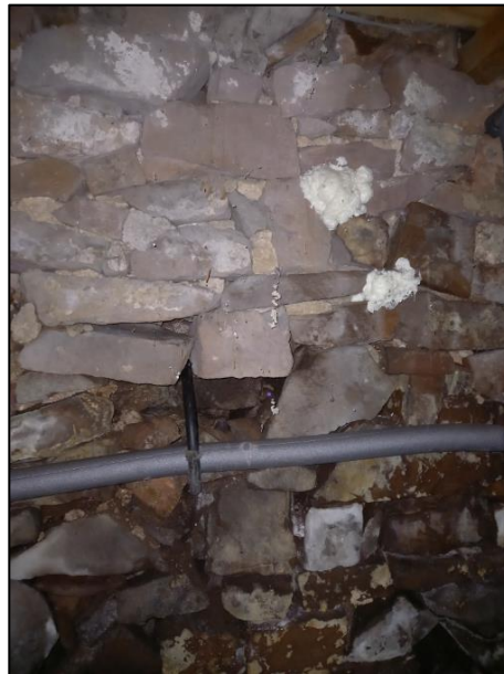
Plate 14: Photograph showing a typical view of the internal stone walls within the northern-most section of the building.
