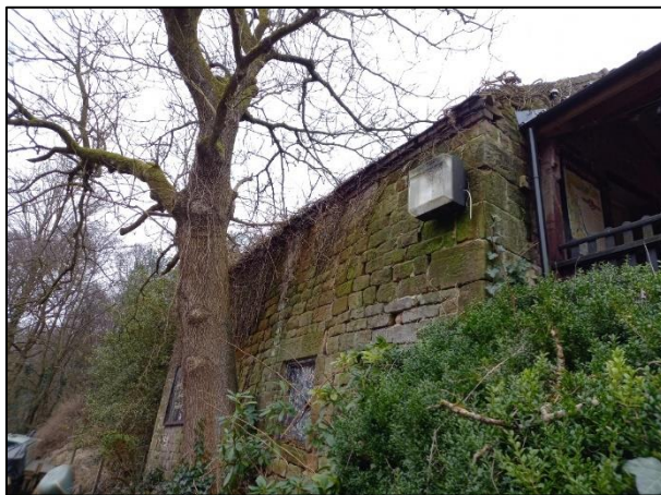
Plate 8: Photograph showing the mature oak tree along the eastern elevation of the building. Photograph facing north-west.
