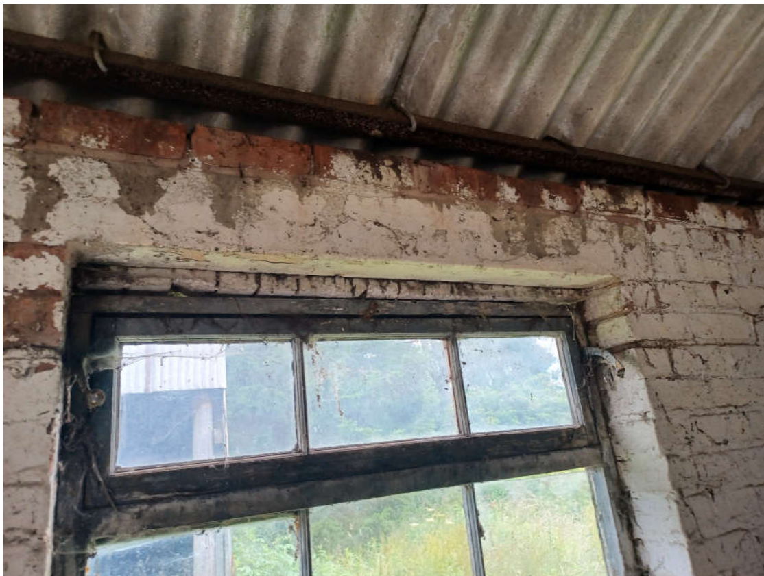
Photo 13 typical lintel to internal leaf of brickwork
