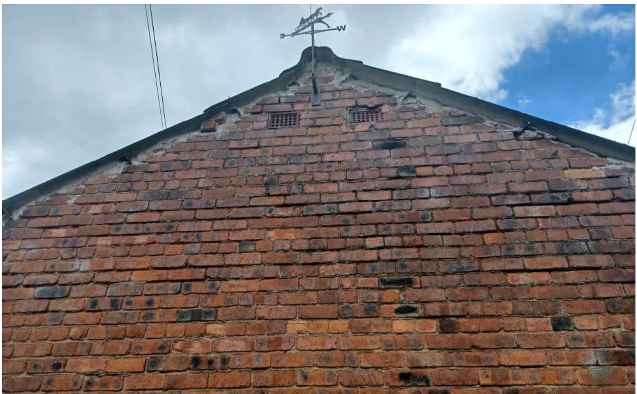
Photo 6 Verge to left hand gables
