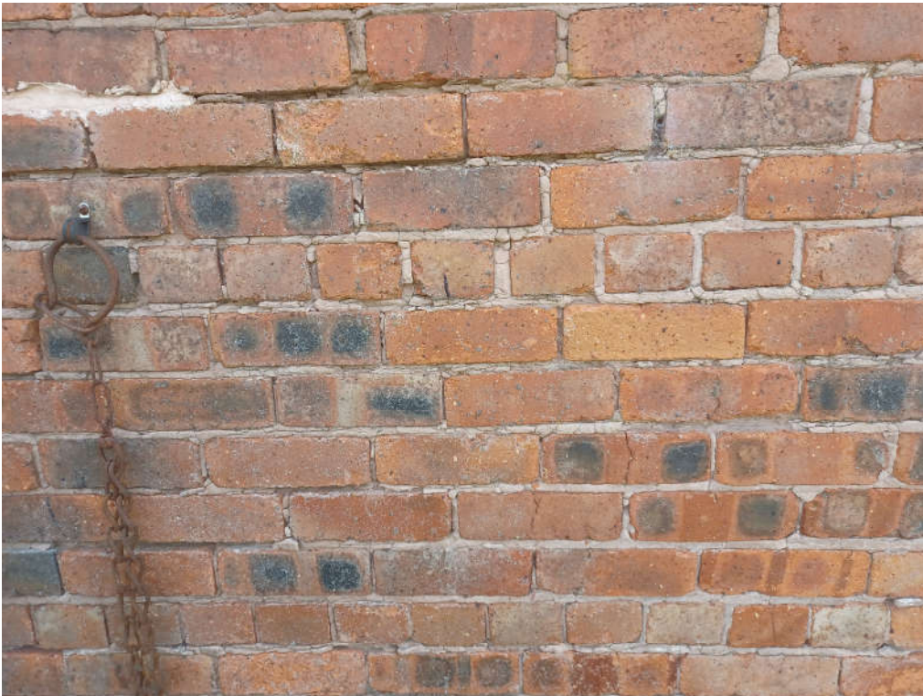
Photo 4 Front elevation brickwork
