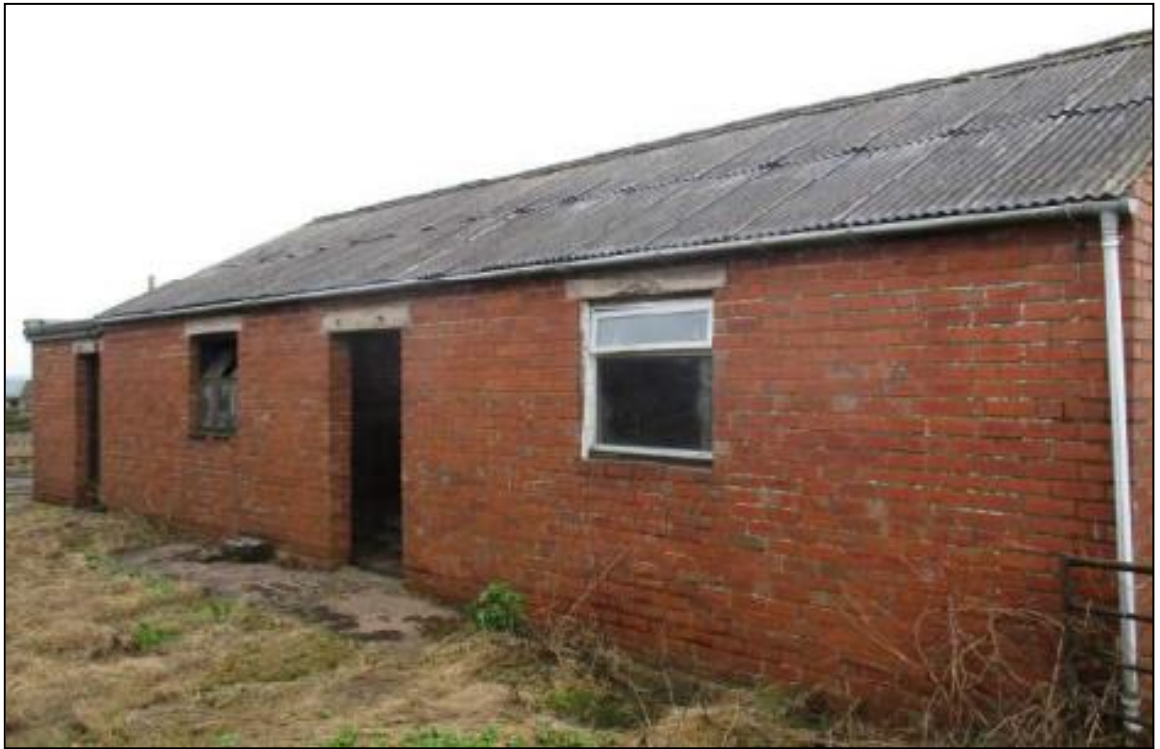
Image 2 – Existing Building at Harveys Lane, Kingsley Moor
