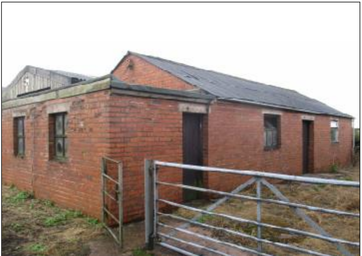
Image 1 – Existing Building at Harveys Lane, Kingsley Moor
