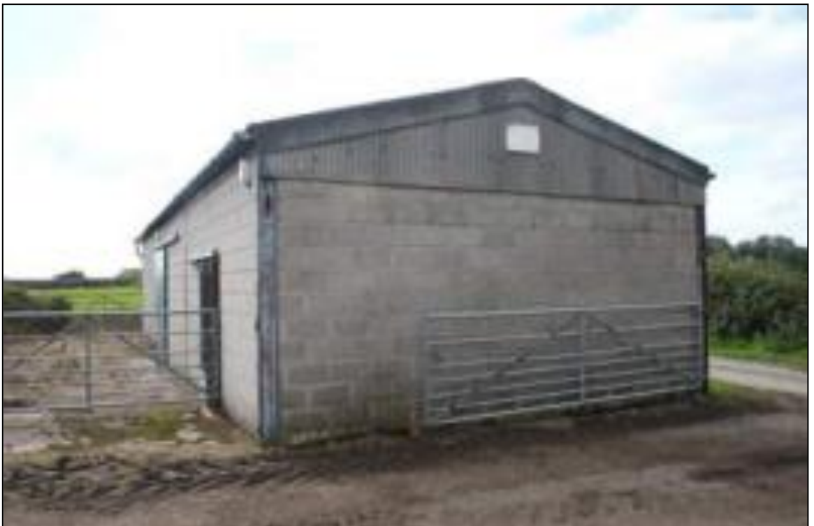
Image 3 – Existing Blockwork Building at Harveys Lane, Kingsley Moor
