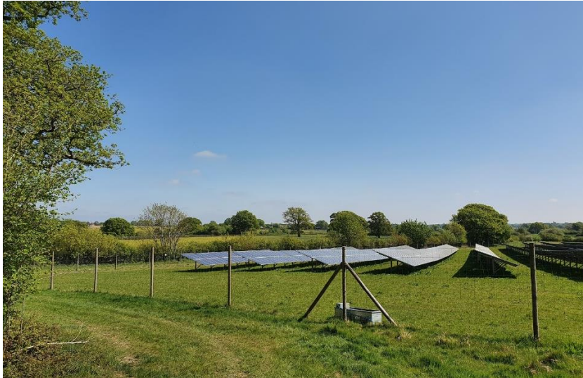
A typical solar array and post and wire deer fencing
