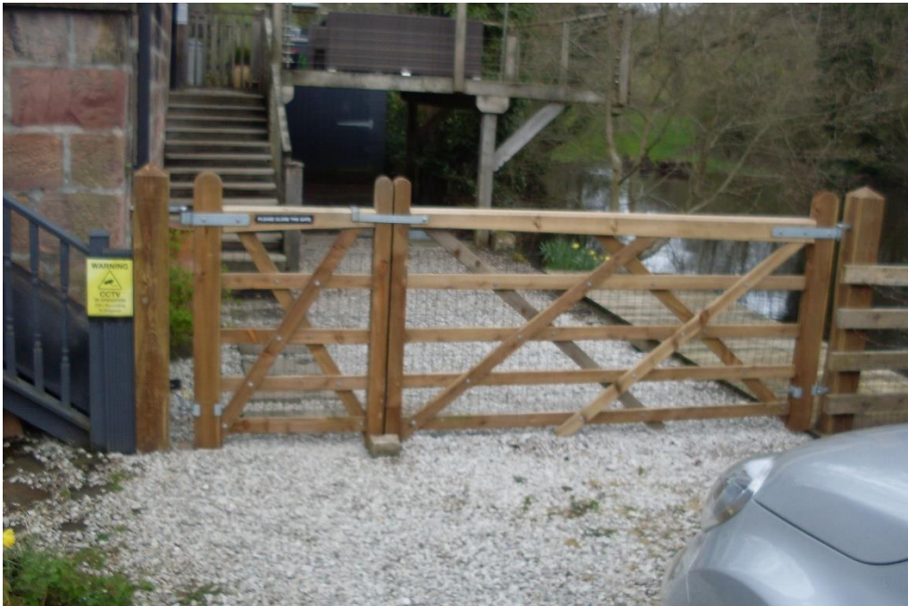
5. Existing timber gate next to house.
