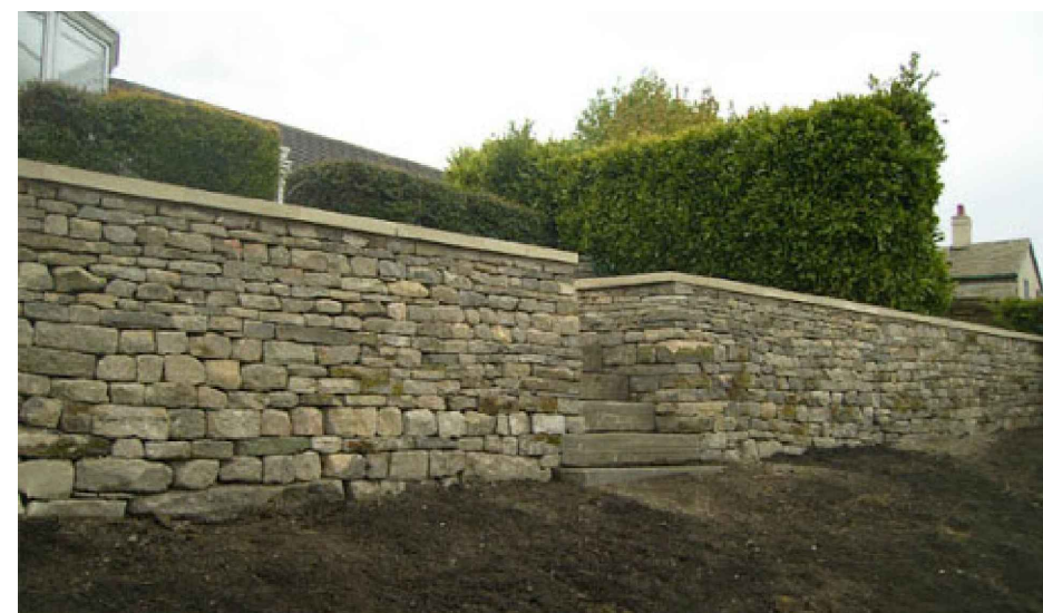
(B) - New Stone Retaining wall
