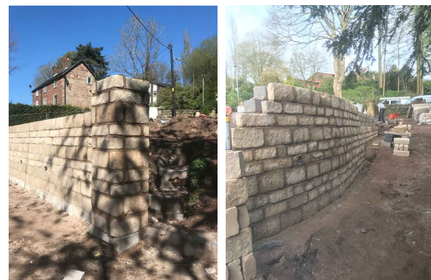
(B) - New Stone Retaining wall
