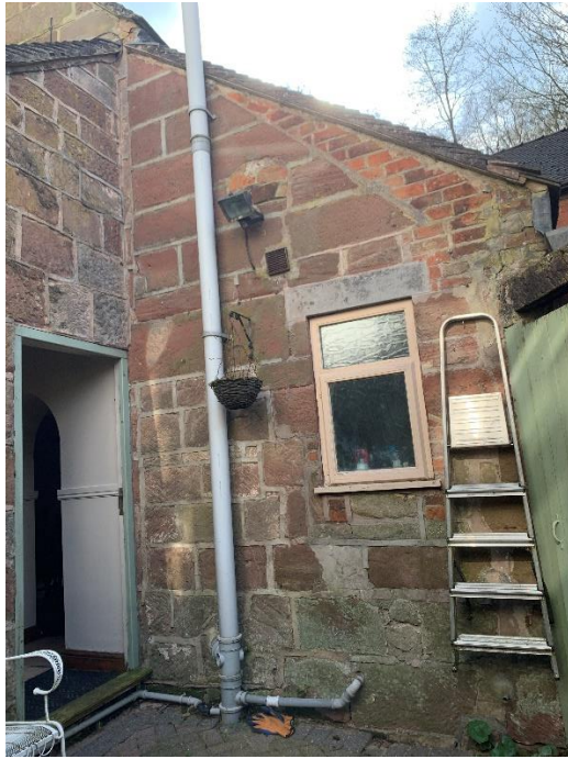
Figure 2 Rear elevation showing existing soil vent pipe
