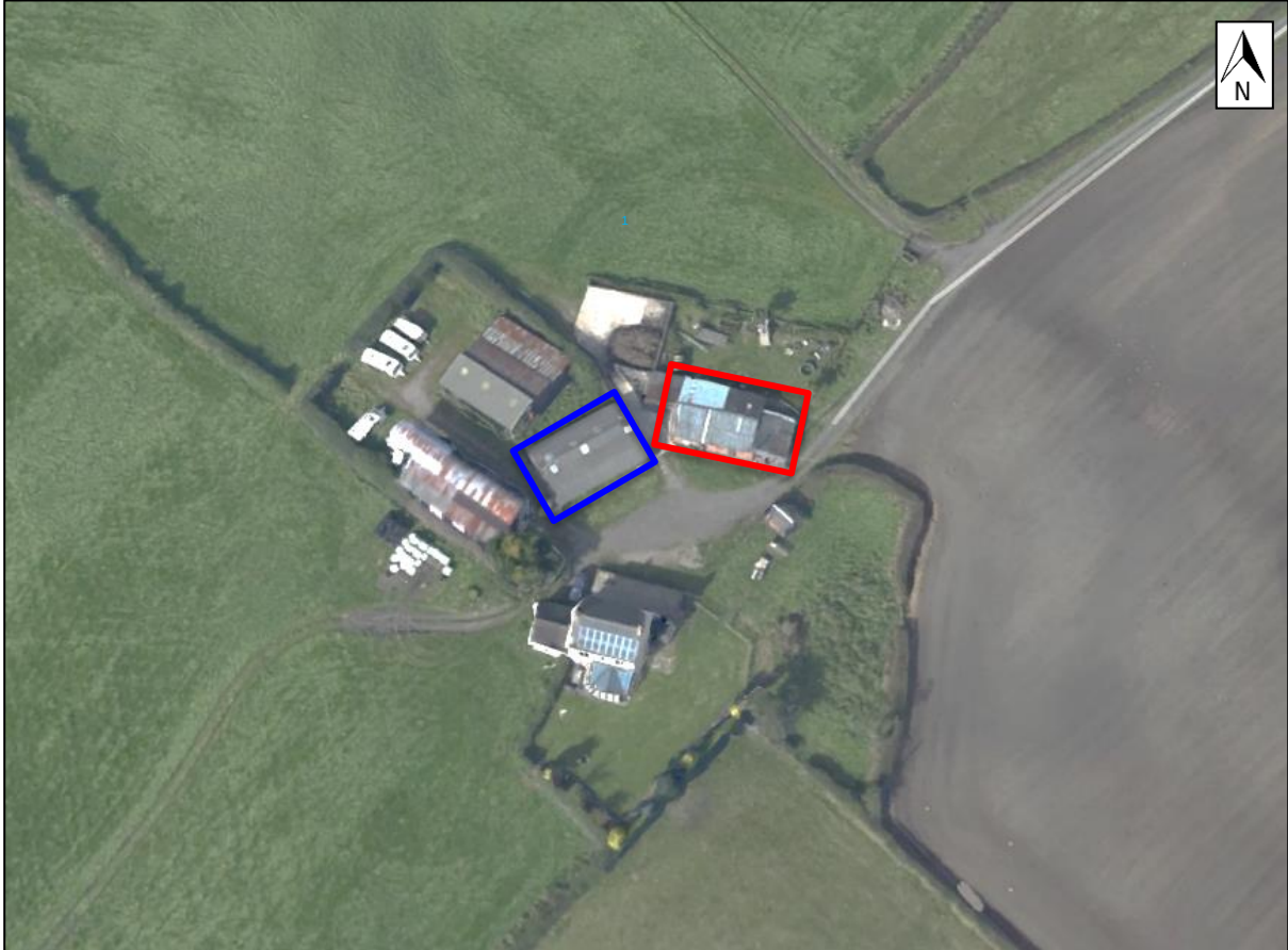
Figure 1: An aerial map showing the surveyed buildings at the 'Old Engine Farm, Dilhorne' in relation to some of the local landscape. The former Milking Parlour is highlighted within the red outline with the adjacent barn highlighted in blue.
