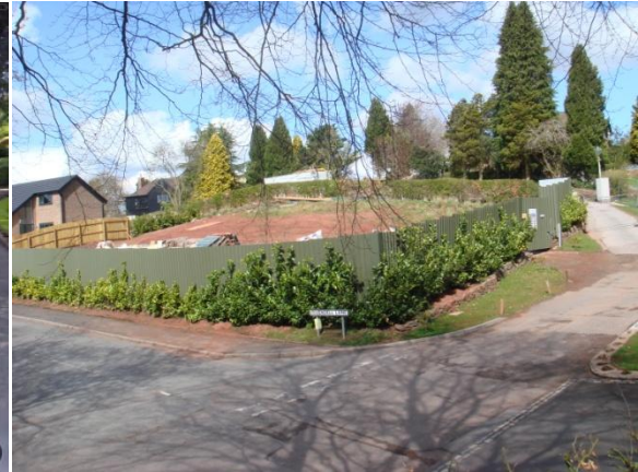
Current site view and levels
