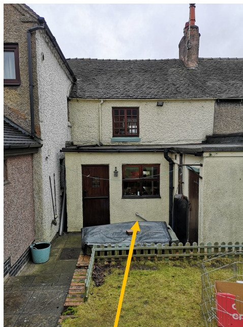
No 2 Church Terrace – Rear Elevation
