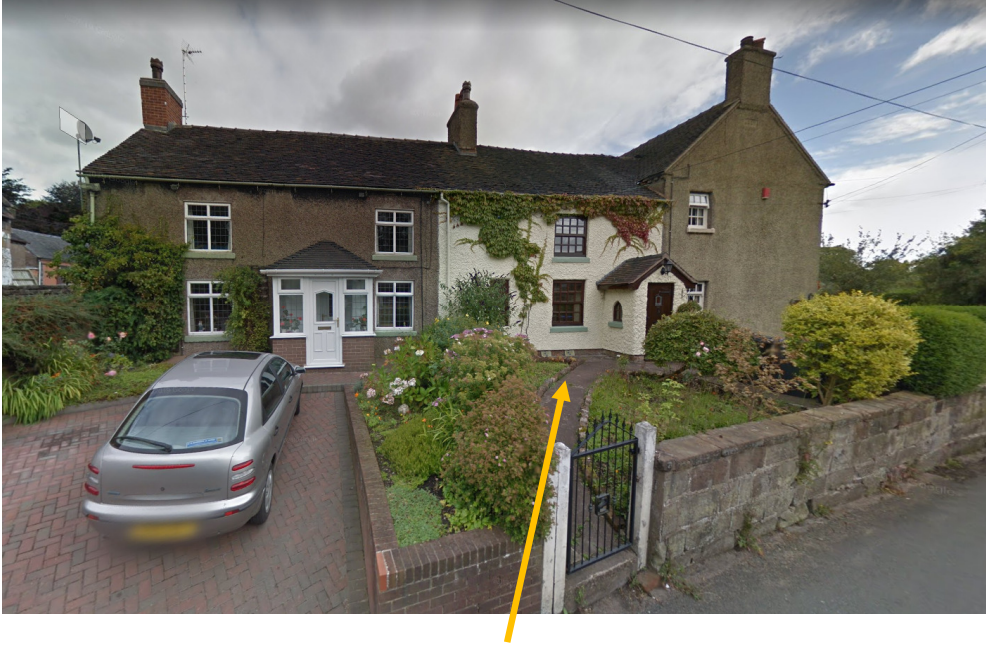
No 2 Church Terrace – Front Elevation
